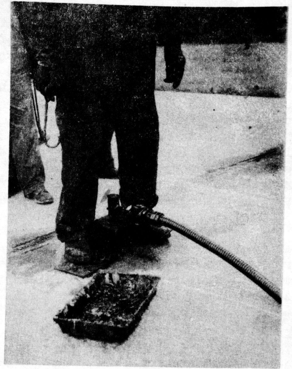
FIGURE 3. NOZZLE FOR PUMPING BITUMINOUS MATERIAL BENEATH THE PAVEMENT.
