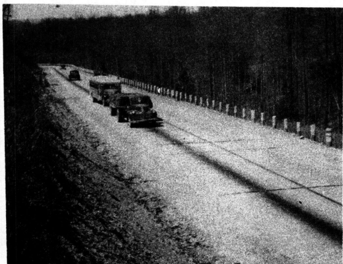
FIGURE 3. NOTE THE DIFFERENCE IN THE OIL STREAKS RESULTING FROM DIFFERENCE IN UP-HILL AND DOWNHILL SPEEDS AND TRACTIVE RESISTANCE OF VEHICLES ON A LONG GRADE. FAP 486 A (2) STA. 380 COFFEE COUNTY (4-6-44)
