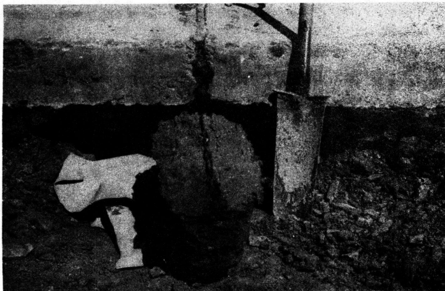
FIGURE 2. UNDISTURBED COLUMN OF SOIL REMOVED FROM UNDER A PUMPING EXPANSION JOINT. NOTE THAT A SOFT MUD HAD FORMED ONLY UNDER THE FAR SIDE OF THE JOINT IN THE DIRECTION OF TRAFFIC.
