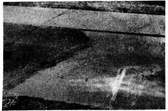
FIGURE 18. THIS IS A VIEW OF THE FIRST CRACK PAST THE JOINT IN FIGURE 17.
