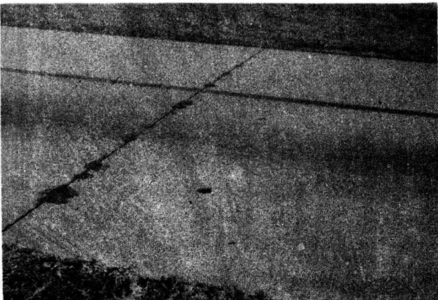
FIGURE 15. A SLAB TREATED WITH MIX "B" THAT HAS GIVEN TWO YEARS OF GOOD SERVICE.
