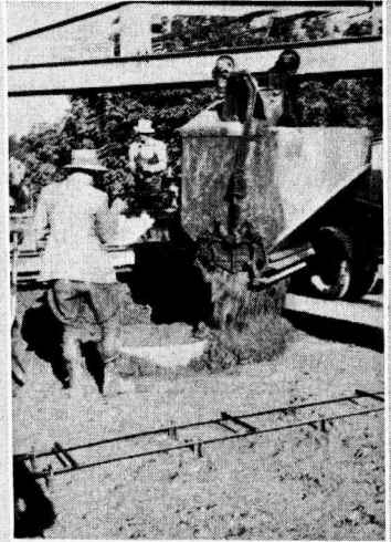
Placing concrete around form.
