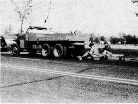
Figure 3. Truck Used Singly for 10,000-lb. Test Reaction - Minnesota
