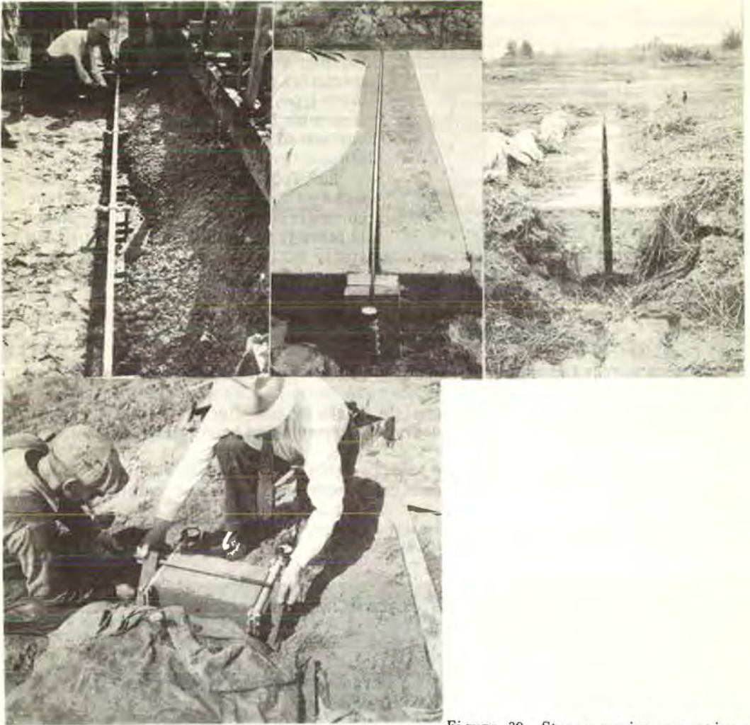
Figure 39. Stress curing operations.
