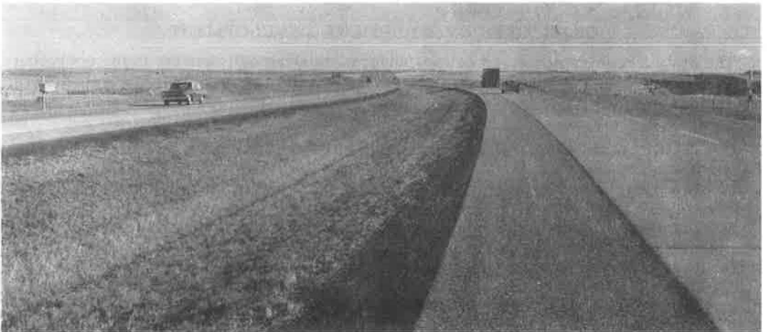
Figure 1. Automatic traffic counter station, Interstate 94.
