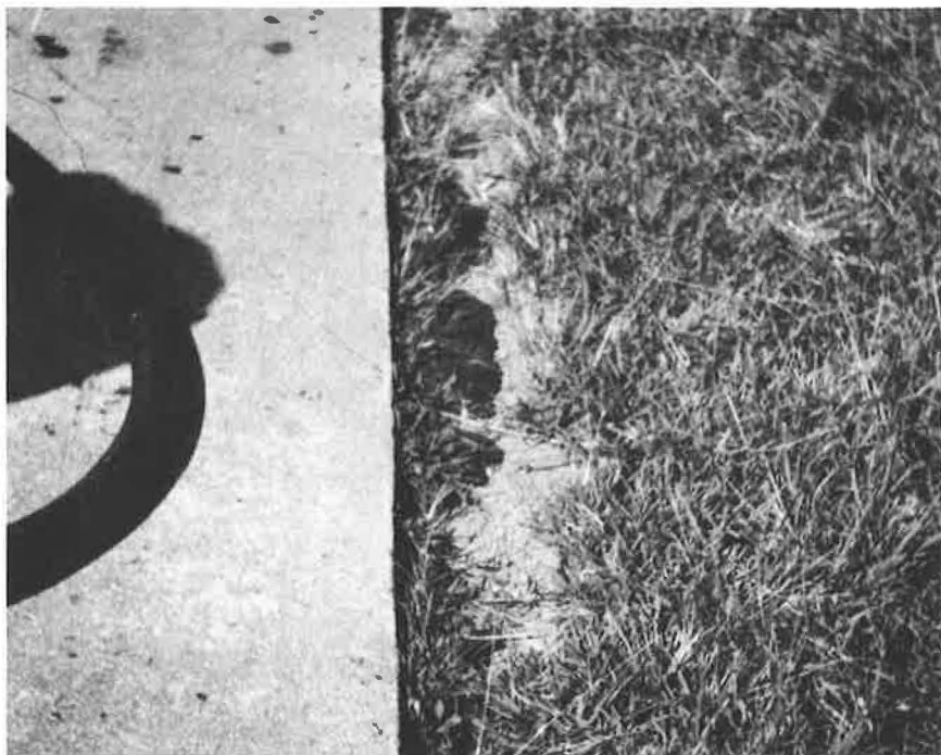
Figure 4. Undiluted Subsealer II being exuded from edge of pavement.
