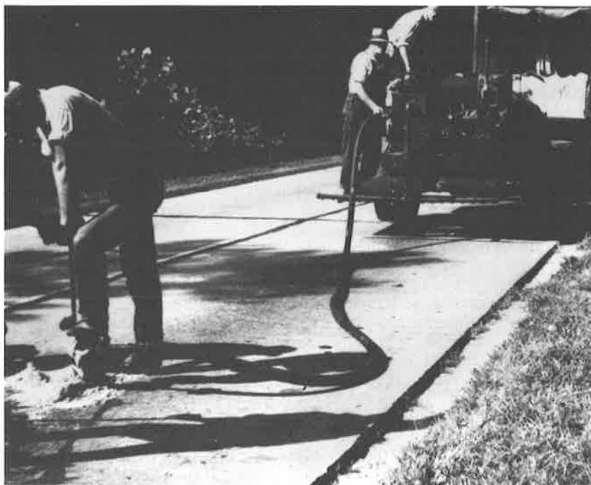
Figure 2. Pumping of subsealer.
