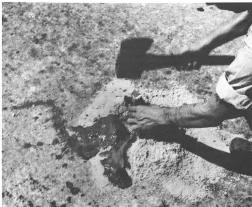
Figure 3. Wooden plug being driven into slab.
