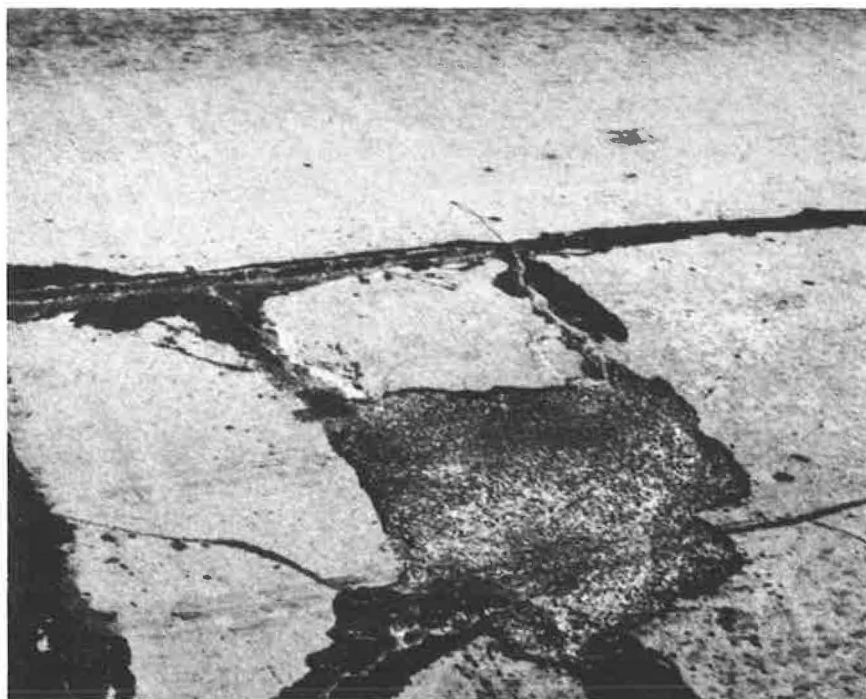
Figure 5. Road with subsealer.
