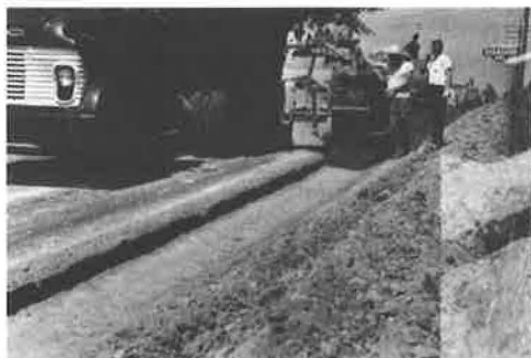
Figure 3. Specially constructed spreader for widening.
