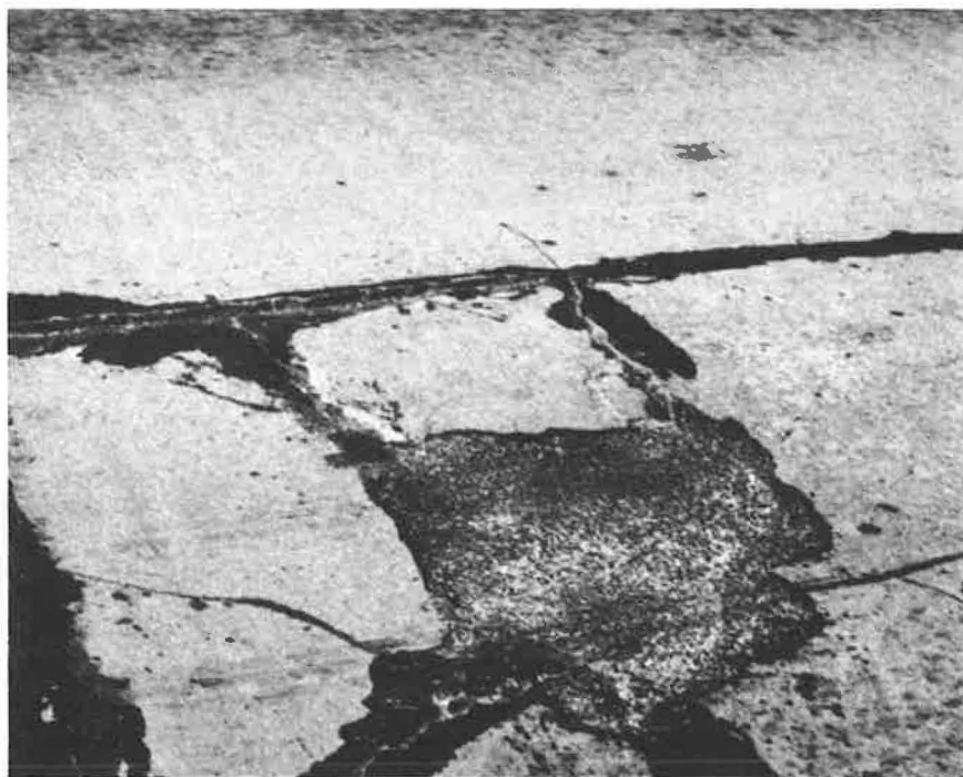
Figure 5. Road with subsealer.
