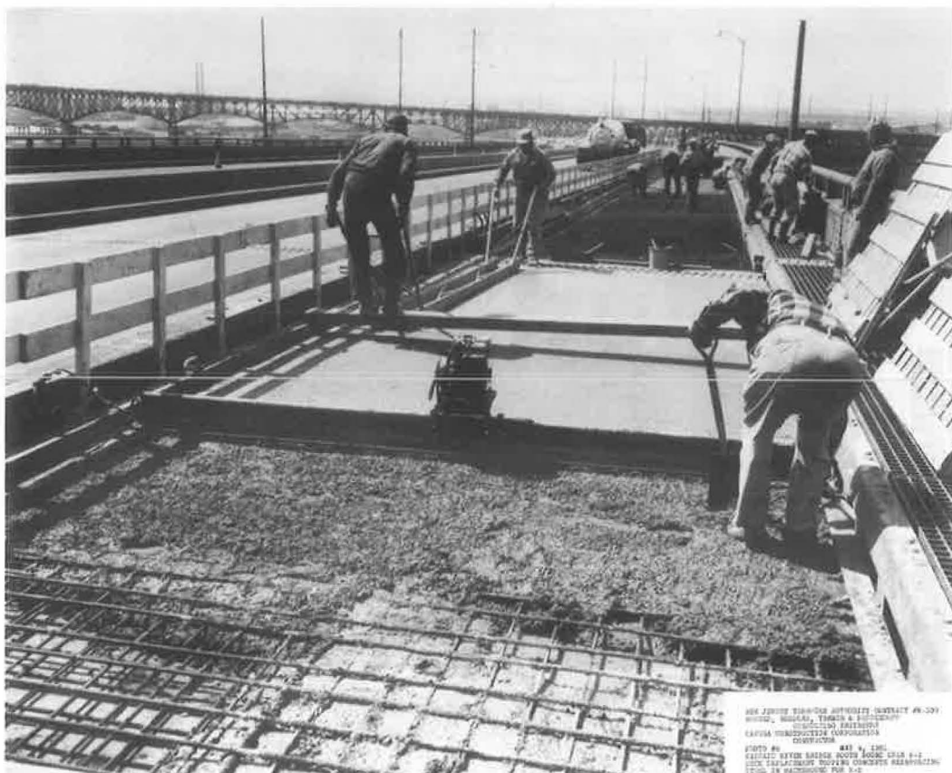
Figure 5. Nonshrinking concrete being placed over fresh conventional concrete.
