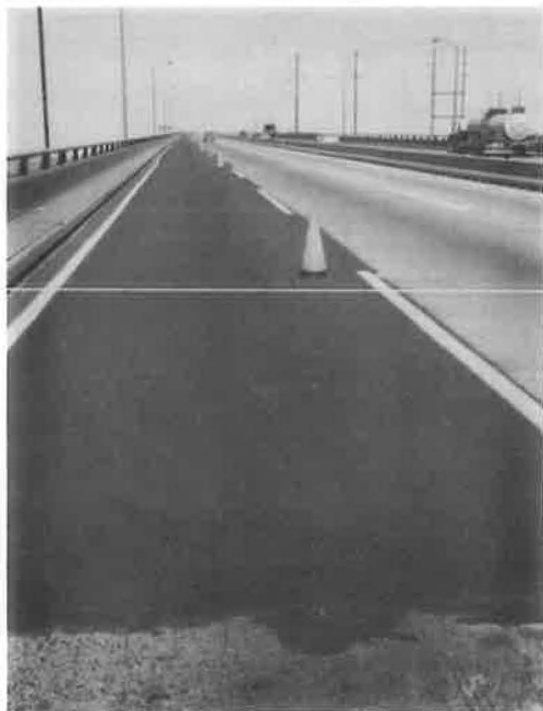
Figure 10. Coal-tar epoxy resin roadway surfacing.
