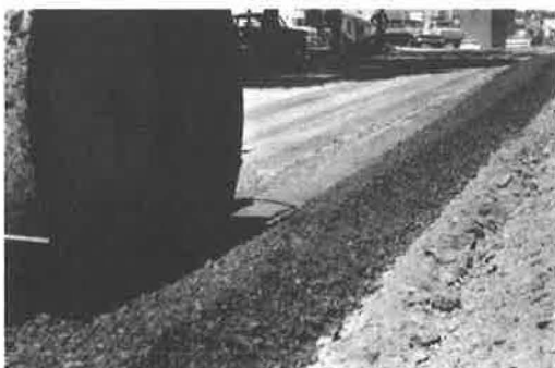
Figure 5. Rerolling surface to finished grade.
