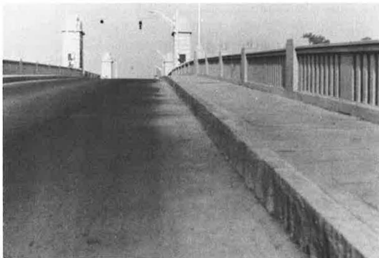
Figure 6. 112th St. Bridge, Troy, after repair; new roadway slab and steel grating on bascule span, new granite curbs, sidewalks repaired and protected by epoxy bonding compound covered with silica sand for traction, all concrete repaired and waterproofed.
