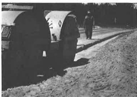
Figure 2. Compacting trench subgrade.
