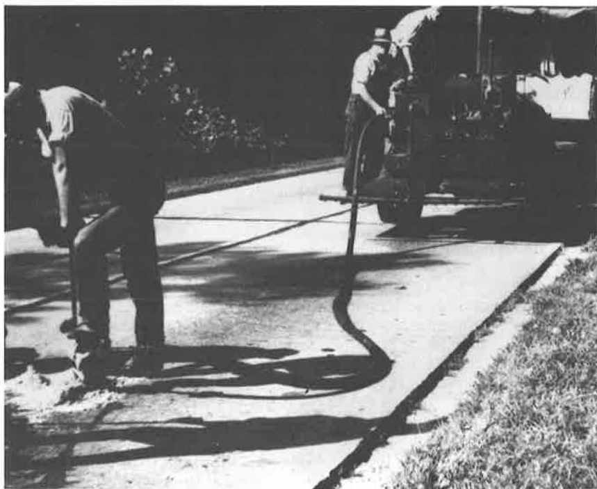
Figure 2. Pumping of subsealer.
