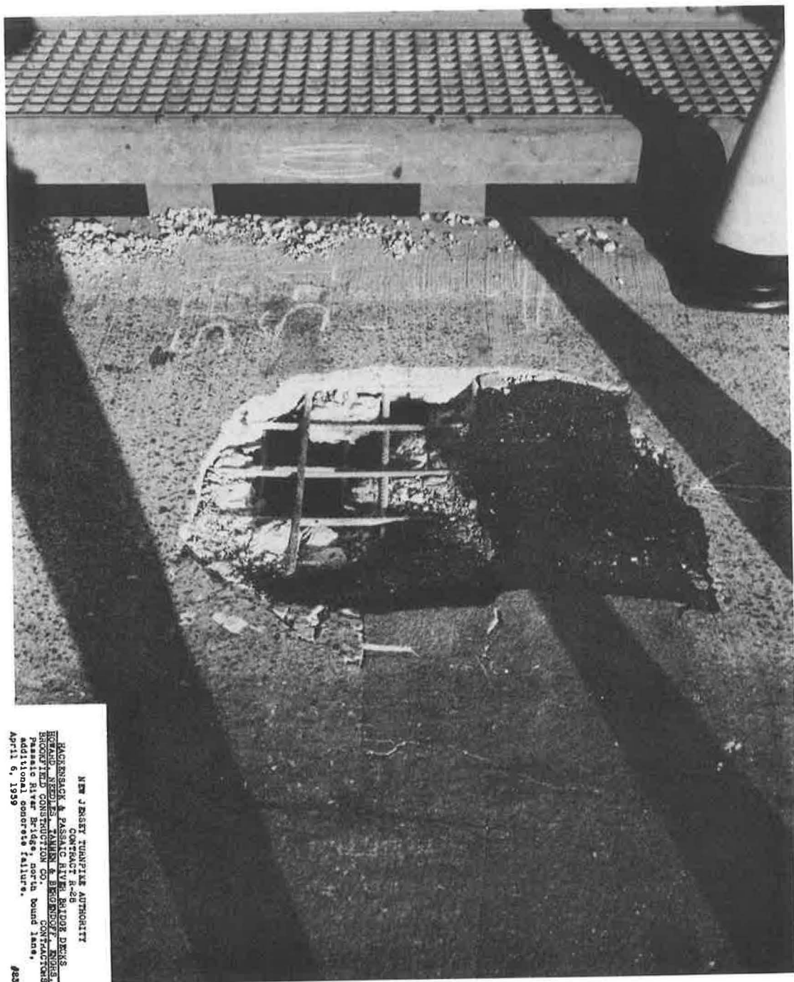
Figure 4. Slab failure.
