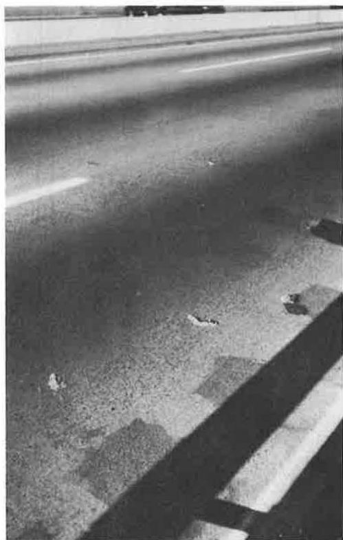
Figure 1. First stage spalling.
