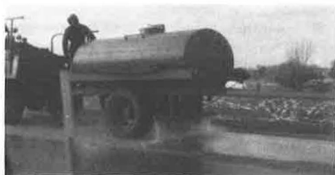
Figure 4. Applying water to ice road.
