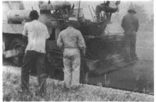
Figure 7. Placing hot asphaltic binder.
