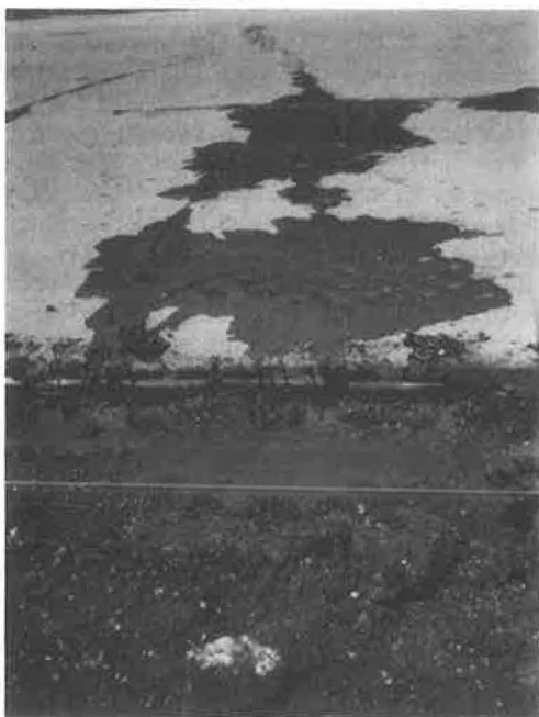
Figure 5. Wet material removed by roller from subgrade under slabs broken by traffic; removed mud in trench.
