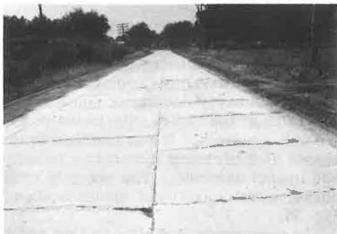
Figure 3. Old roadway showing pumping under normal traffic; 3-ft base widening in place, before any breaking and seating operation.
