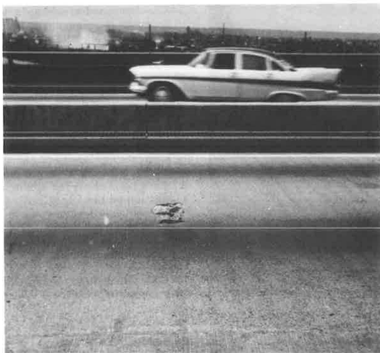
Figure 2. Second stage spalling.
