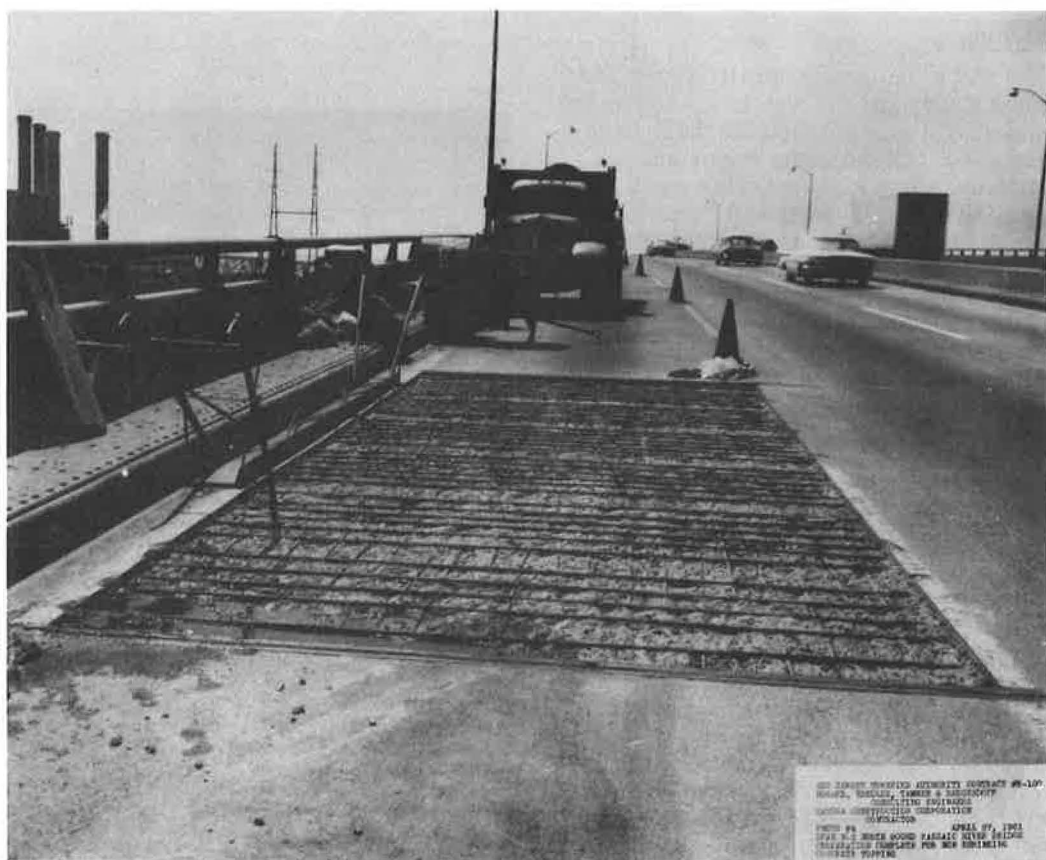
Figure 6. Excavated surface ready for nonshrinking concrete topping.
