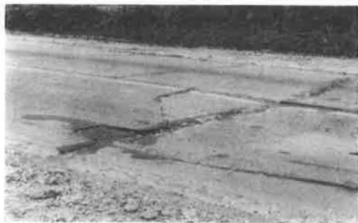
Figure 1. Old, broken, and rough rigid pavement.
