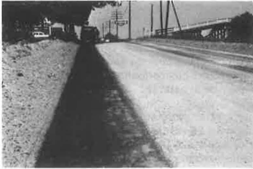
Figure 6. Bituminous prime coat.
