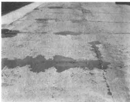
Figure 4. Wet material displaced by rolling at typical pumping slabs.
