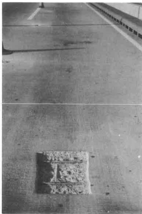
Figure 7. Pothole well prepared for patching.
