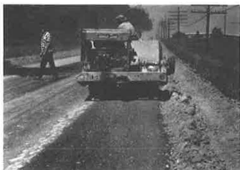
Figure 4. Compacting mixture.
