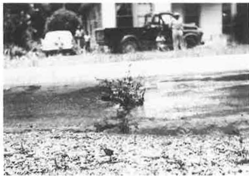
Figure 1. Typical slab pumping under truck traffic on old roadway before construction.
