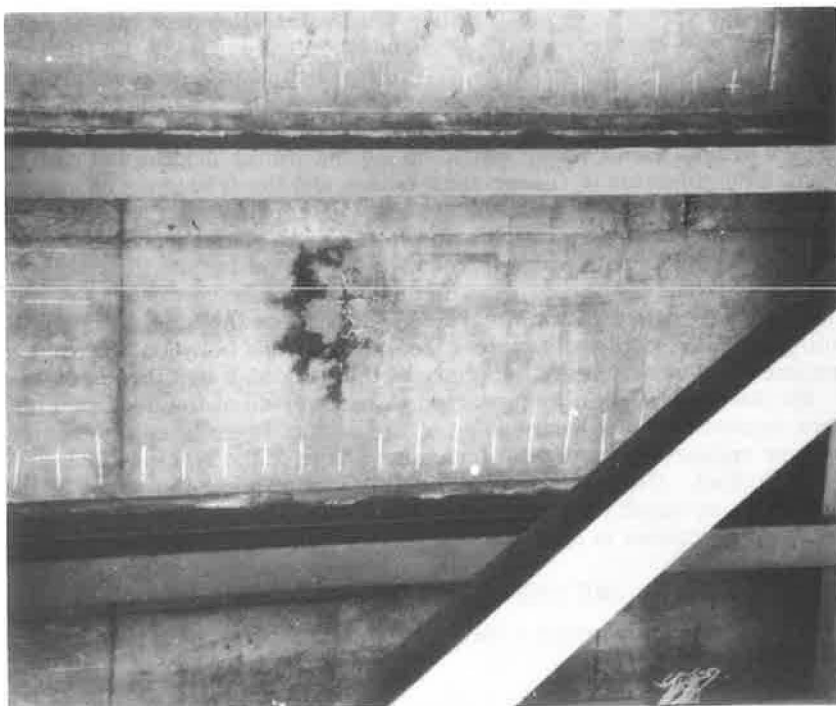
Figure 3. Underside checkerboard cracking.
