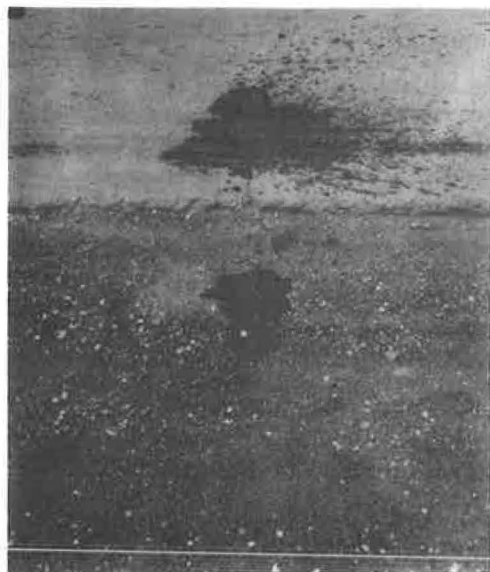
Figure 6. Wet subgrade material forced through shoulder by roller.
