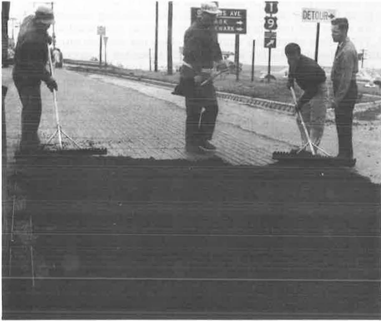
Figure 6. Spreading sand-mix asphalt.
