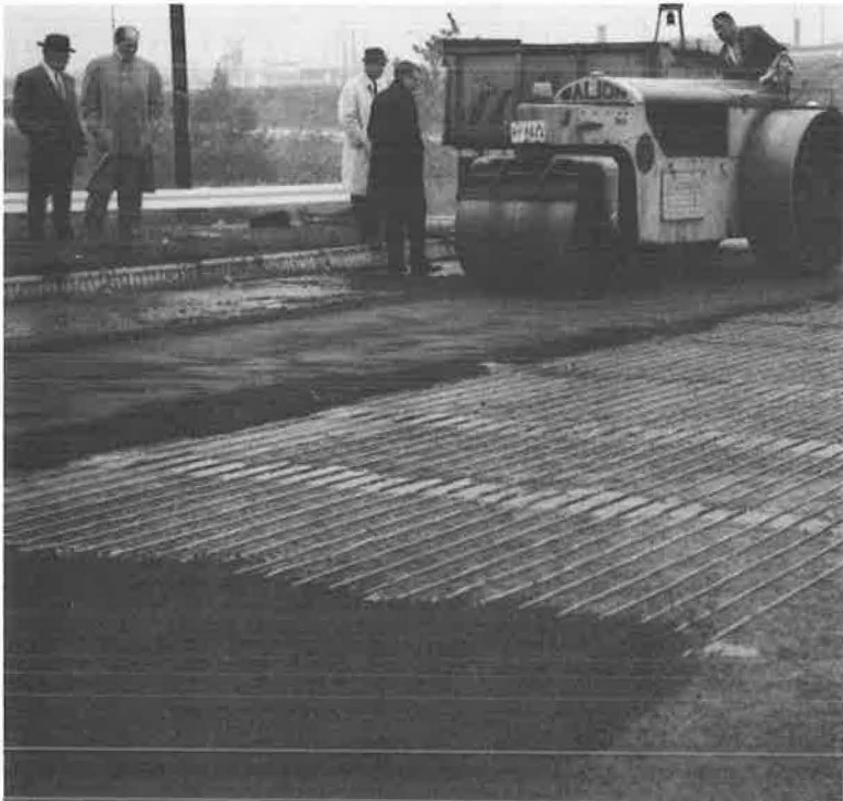
Figure 7. Rolling sand-mix.
