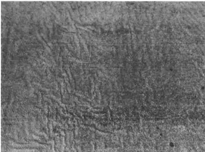
Figure 2. Polyester mortar overlay on PCC surface.
