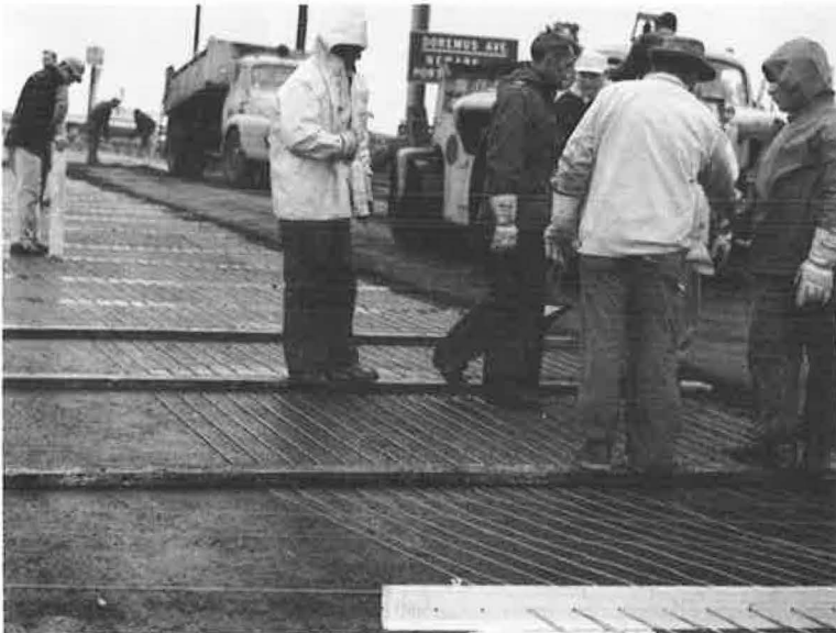
Figure 4. Laying cable, land fill area.
