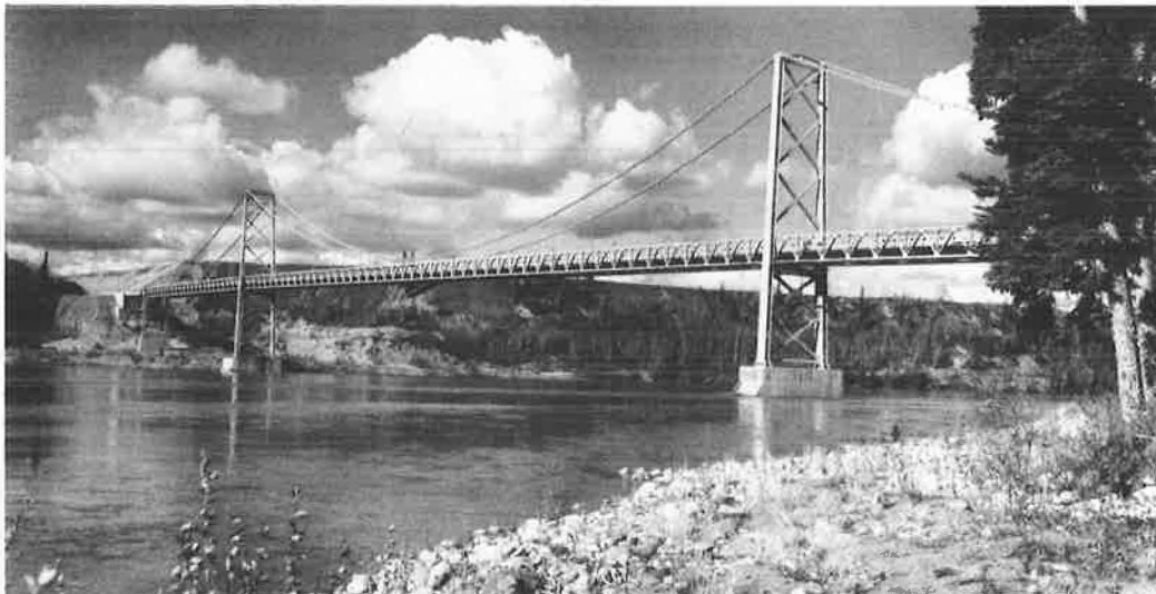
Figure 1. The Peace River highway bridge as originally constructed.
