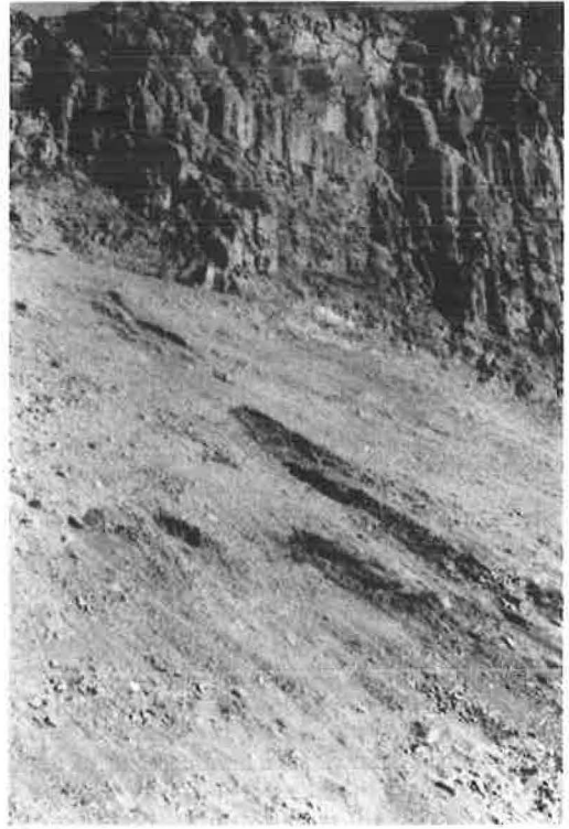
Figure 10. Bouldered layer on surface in Fig. 9 stripped off, showing segregated strata deposited flatter than angle of cut slope.
