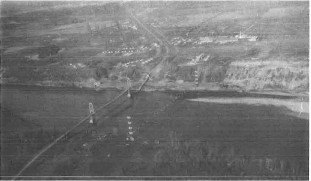
Figure 2. Gas processing plant and pipeline suspension bridge in relation to highway bridge.
