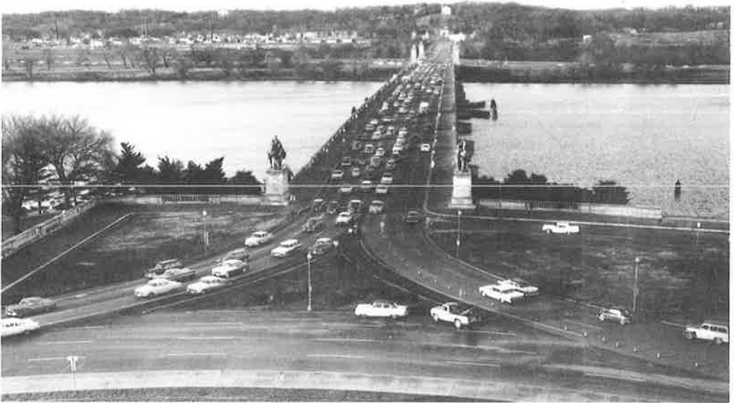
Figure 11. More uniform distribution of morning traffic in the four inbound lanes, Memorial Bridge.
