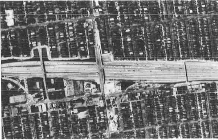
Figure 3. Aerial view, Congress-Harlem interchange.
