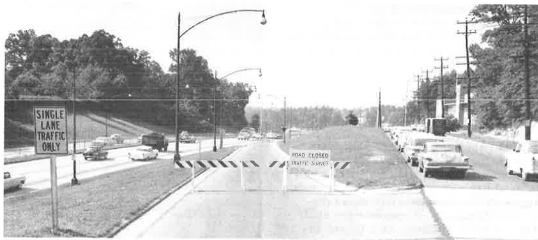
Figure 3. Method of closing 10th Street northbound on-ramp, viewed from Williams Street.
