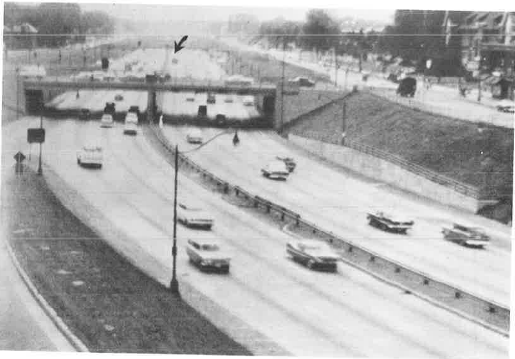
Figure 3. Median lane closure, Gladstone, after phase.
