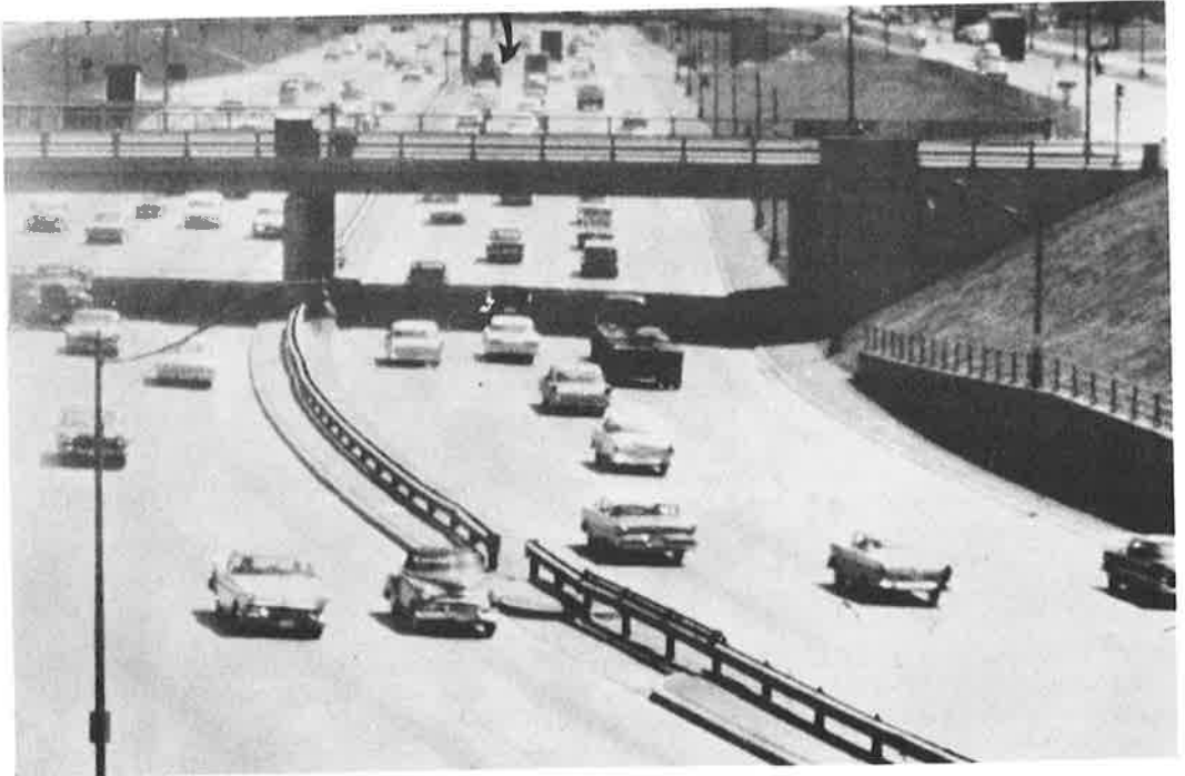
Figure 2. Median lane closure, Gladstone, before phase.
