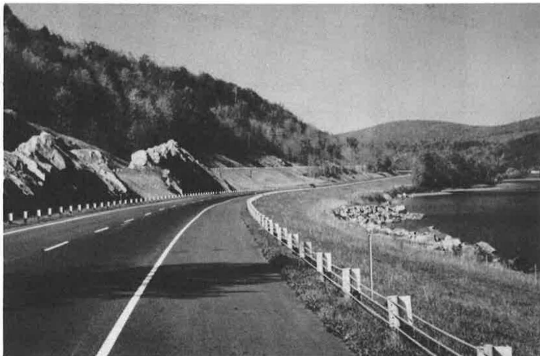
Figure 4. Integration with the landscape: Massachusetts Turnpike around Greenwater Lake. Notable are the relationship to both water and hill, the sculptural use of rock outcrops, and the treatment of existing vegetation.
