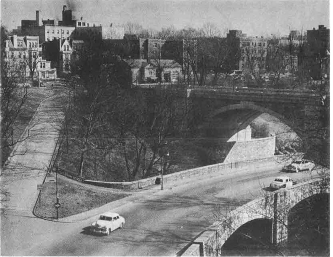
Figure 2. Typical area on Rock Creek Parkway for sludge application.
