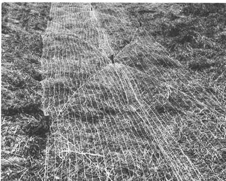
Figure 2. Pegs hold paper netting in place over mulch. Staples and stapling guns can be used to fasten netting instead of driven stakes and twine.
