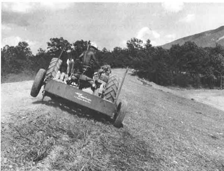
Figure 1. An anchoring tool being used effectively to tie down mulch on a watershed project.
