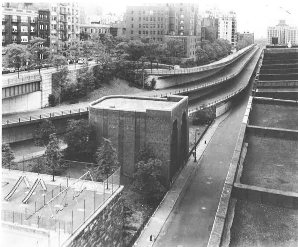
Figure 2. Integration with the environment: an imaginative solution under congested urban conditions (Interstate 278 in Brooklyn Heights).
