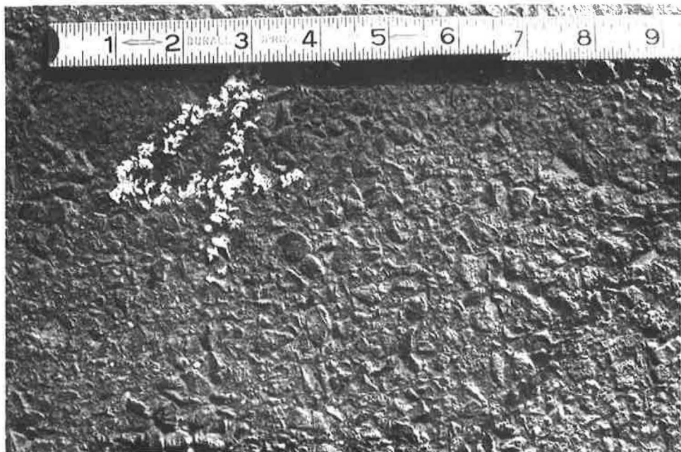
Figure 9. Variations in surface disintegration, North 13th Street, Manville, N. J., August 1962, standard pavement mix.
