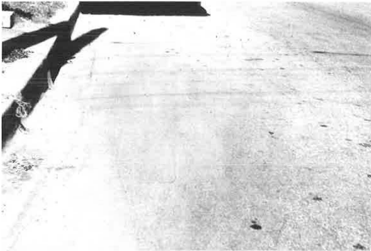
Figure 8. Ross Avenue, Dallas, Texas, August 1962: (top) intersection with Bennett Avenue (map in Fig. 3) with standard mix 5.0 percent asphalt content in foreground and asbestos-modified pavement with 7.5 percent asphalt content at intersection; (bottom) asbestos pavement with 7.5 percent asphalt content at bus stop, opposite corner.
