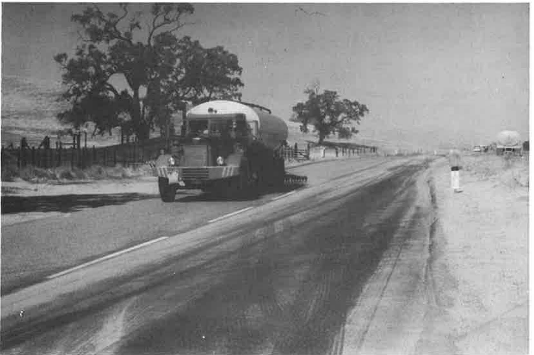
Figure 24. Spraying cationic maltenes emulsion in preventive maintenance; right lane lightly sanded.
