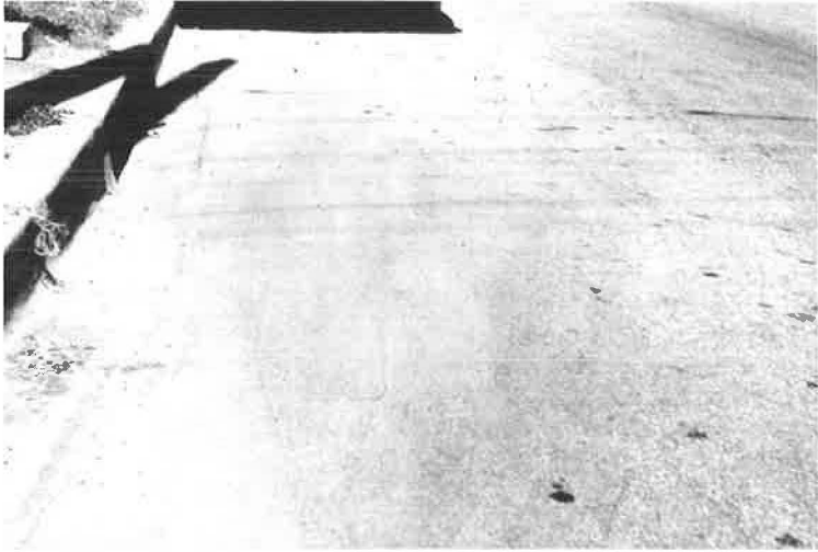
Figure 8. Ross Avenue, Dallas, Texas, August 1962: (top) intersection with Bennett Avenue (map in Fig. 3) with standard mix 5.0 percent asphalt content in foreground and asbestos-modified pavement with 7.5 percent asphalt content at intersection; (bottom) asbestos pavement with 7.5 percent asphalt content at bus stop, opposite corner.
