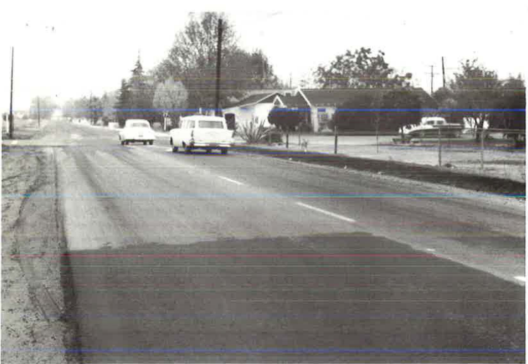
Figure 22. Asphalt section treated with cationic maltene emulsion as construction seal: after rainstorm treated section dried quickly (background); untreated portion retains water in pores (foreground).
