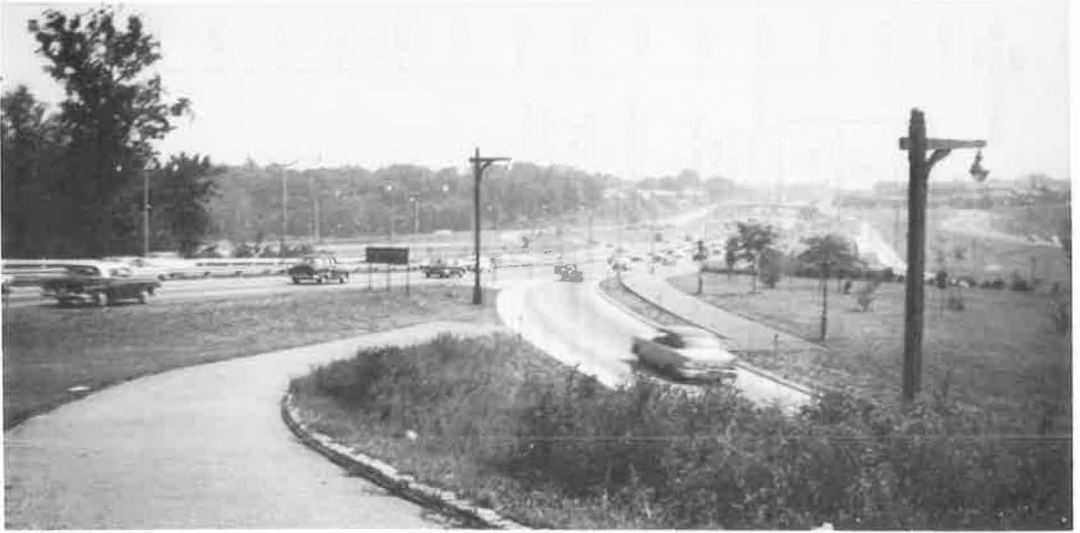
Figure 11. Merging terminal of loop ramp from Cross Island Parkway southbound to Long Island Expressway eastbound on Long Island, N. Y.
