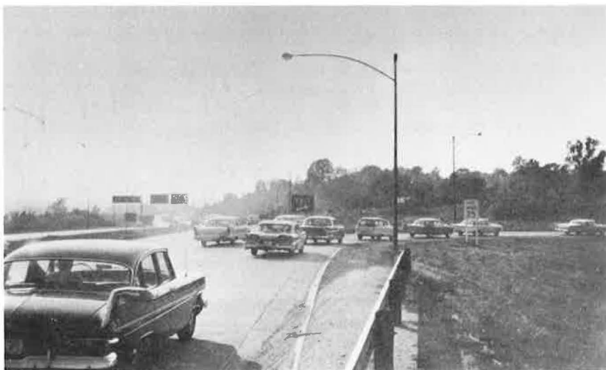
Figure 21. Crowding in at exit nose, illustrating failure to use auxiliary lane to best advantage.
