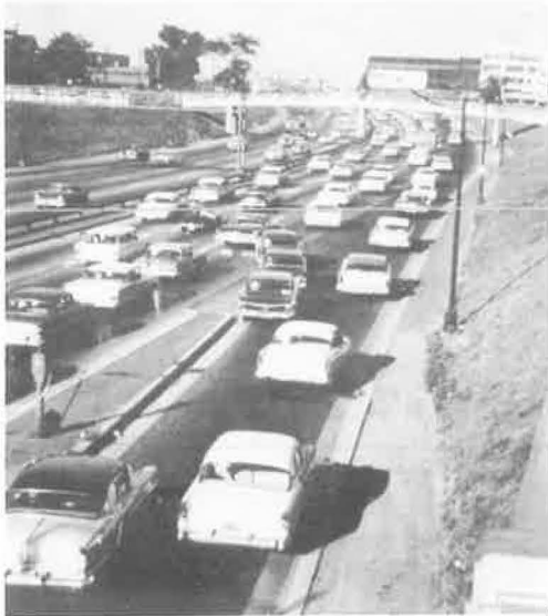
Figure 12. Beaubien ramp to Edsel Ford Expressway eastbound, showing poor operation resulting from 1-lane ramp being pressed into 2-lane service by crowding.
