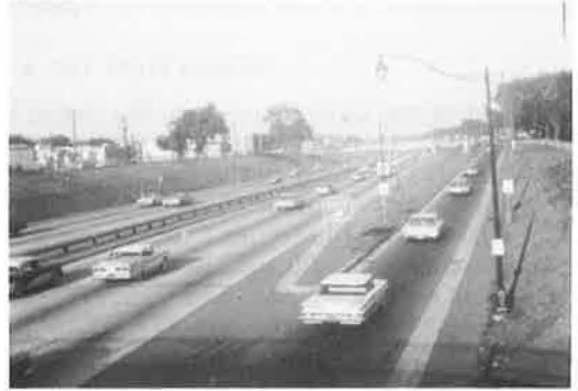
Figure 29. Chalmers exit ramp from Edsel Ford Expressway; volume on expressway upstream from ramp is near possible capacity.
