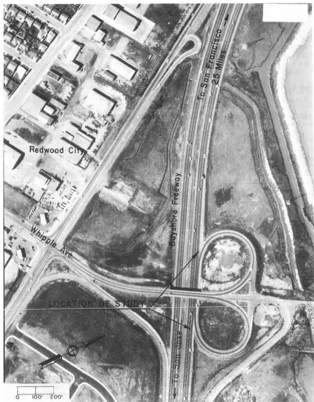
Figure 1. Whipple Ave. Interchange, Bayshore Freeway.
