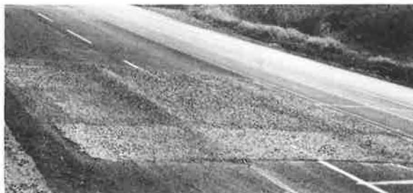
c - General view of rumble strip. Note the alternate dense-graded asphalt plant mix and coarse aggregate rumble sections.
