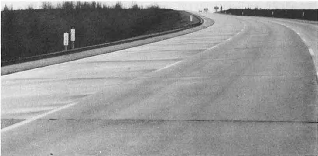
Figure 11. Curled pavement slabs.
