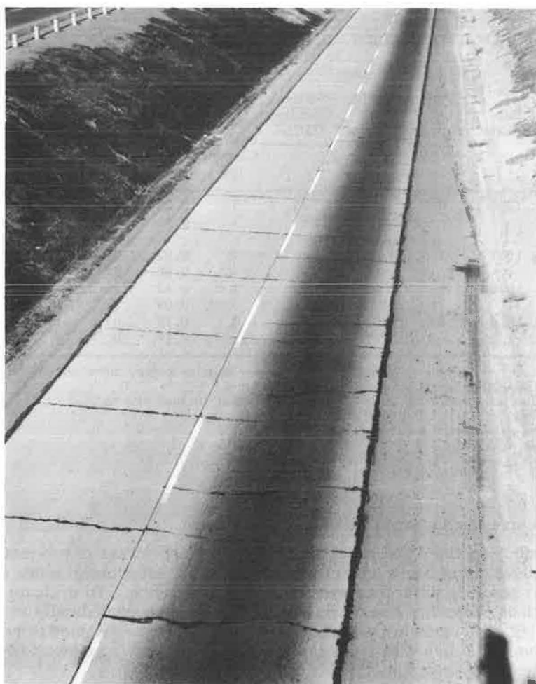
Figure 14. Pavement containing \text{CaCl}_2 , Merced County.
