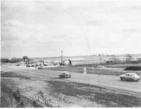
CONDITION 1 - NO CHANNELIZATION
