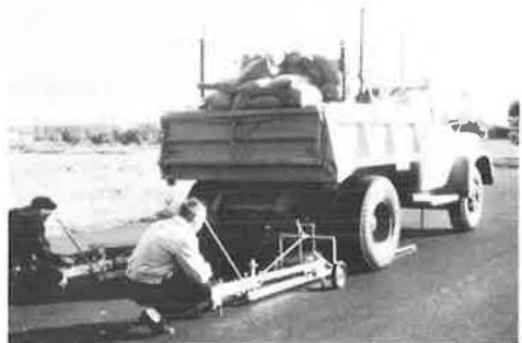
Figure 16. Benkelman beam and truck.
