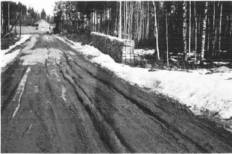
Figure 2. Spring breakup on gravel roads in Central Finland.
