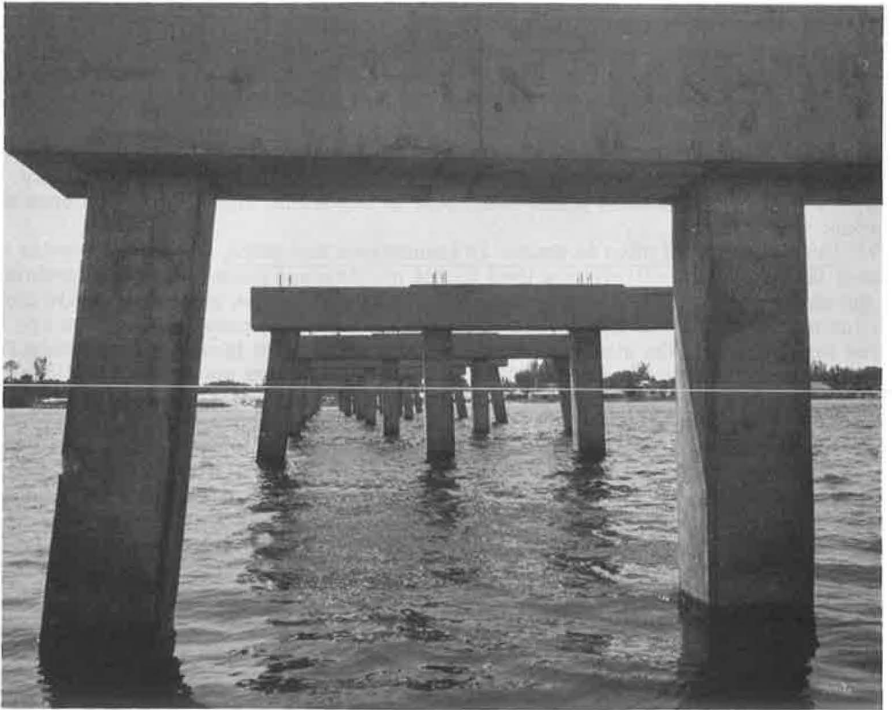
Figure 11. Four 24-in. square prestressed piles extend to provide pier columns for typical Florida crossing.
