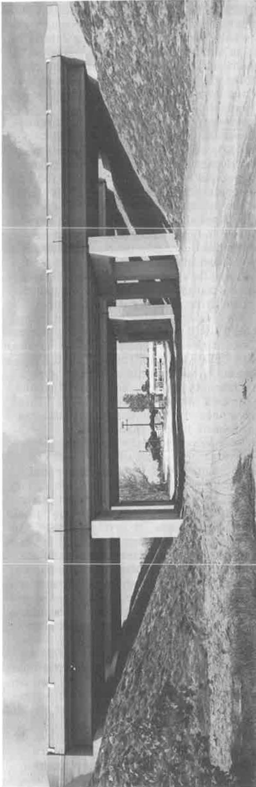
Figure 4. Typical overpass on Sunshine State Parkway, Florida. Structure is a fine example of design simplicity which is a key factor in low-cost prestressed bridges.
