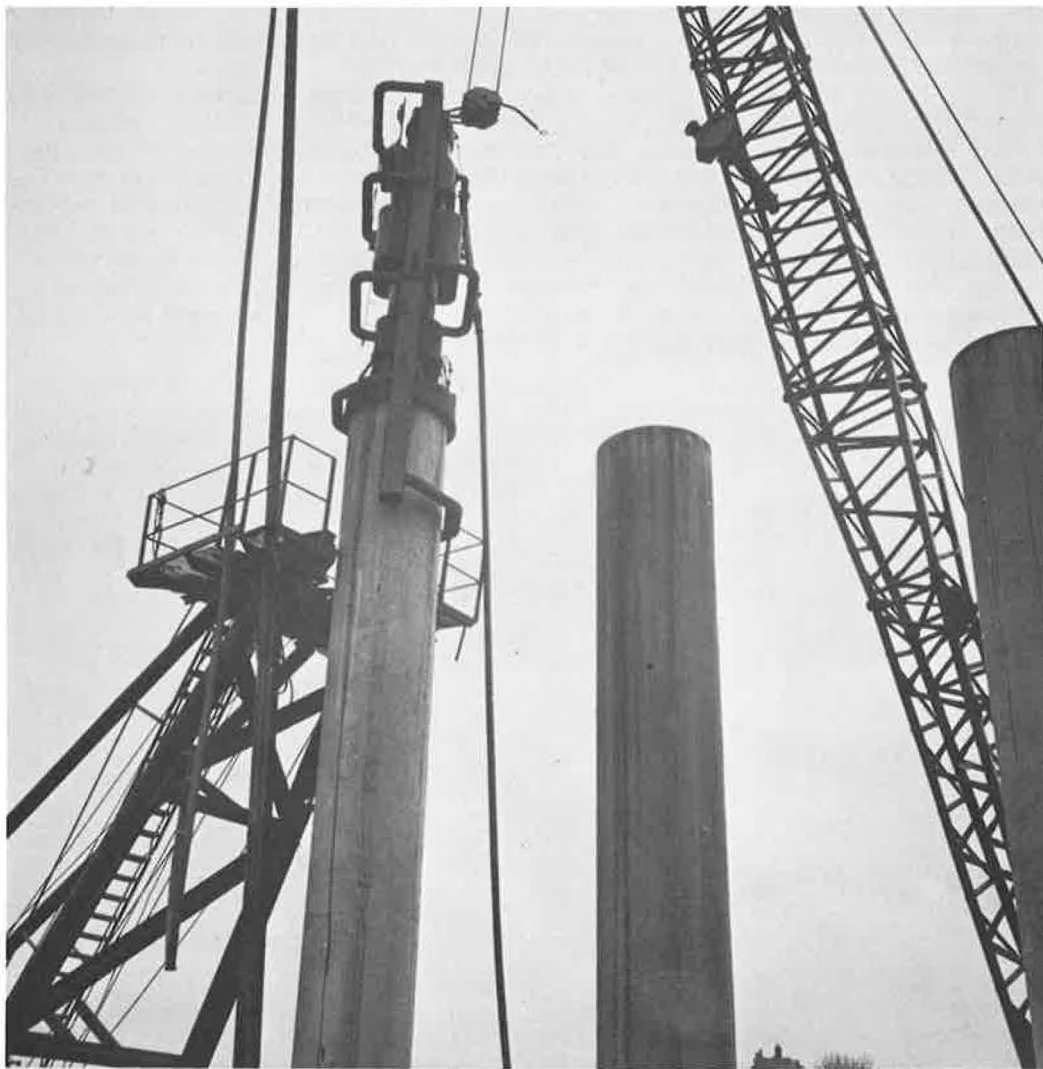
Figure 12. Driving pretensioned cylinder piles for a bridge in Tacoma, Wash.; 48-in. piles driven plumb to act as columns for piers.
