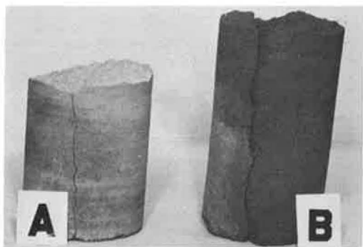
Figure 8. Crack pattern of 4-in. diameter road cores with cement contents of 13 and 7 percent after one year.
