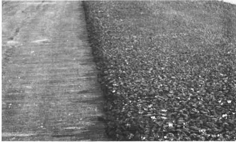
Figure 5. Open textured asphaltic concrete base course, test section B.
