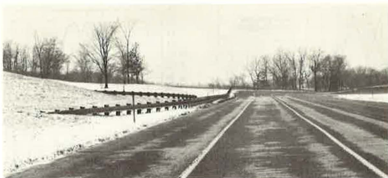
Figure 27. Guardrail buried in back slope and anchored in concrete block.
