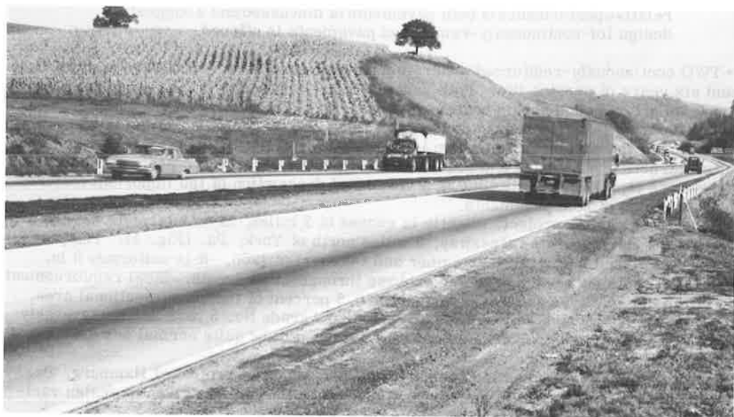
Figure 2. Interstate 78, US 22, Berks County.
