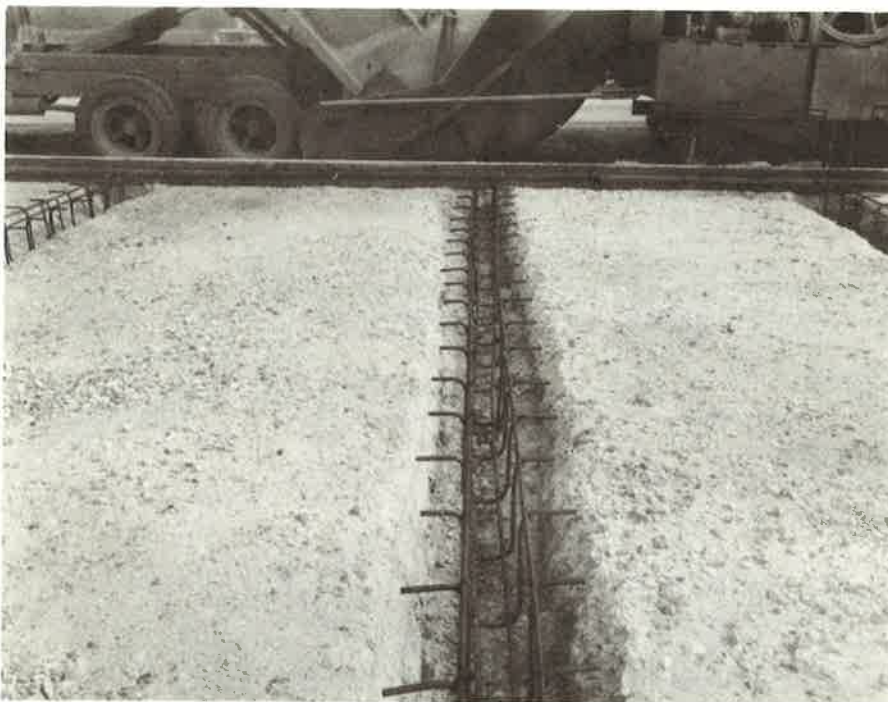
Figure 9. Details of reinforcing steel cage in end restraint lugs.
