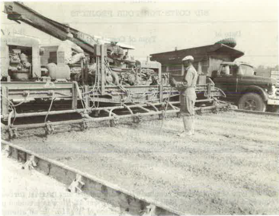
Figure 7. Pavement construction showing internal vibration of concrete.
