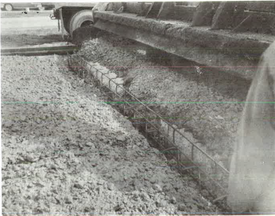
Figure 12. Concrete pouring in vicinity of end restraint lug.
