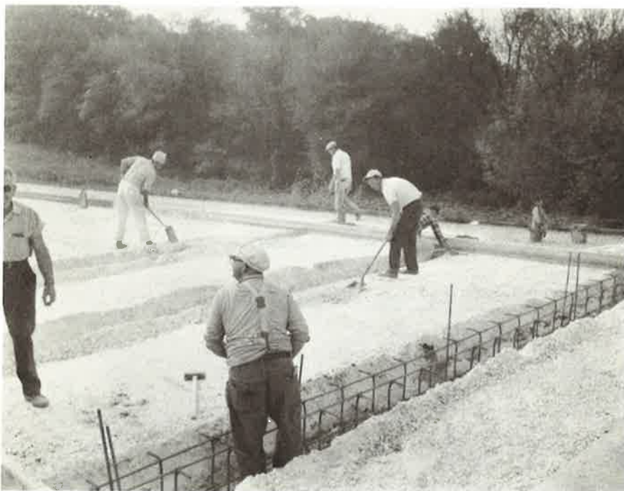
Figure 10. Placing reinforcing steel and trimming subbase at end restraint lugs.
