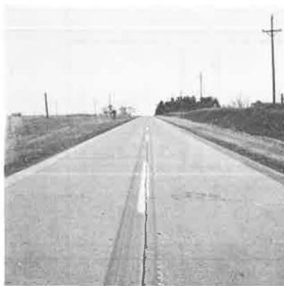
Figure 1. Concrete pavements with satisfactory service: (a) project 52-7, 42 years old, Iowa City stone; (b) project 52-5, 36 years old, Deavenport stone; and (c) project 3-4, 32 years old, Dubuque stone.
