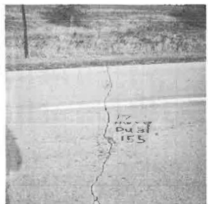
Figure 1. Concrete pavements with satisfactory service: (a) project 52-7, 42 years old, Iowa City stone; (b) project 52-5, 36 years old, Deavenport stone; and (c) project 3-4, 32 years old, Dubuque stone.
