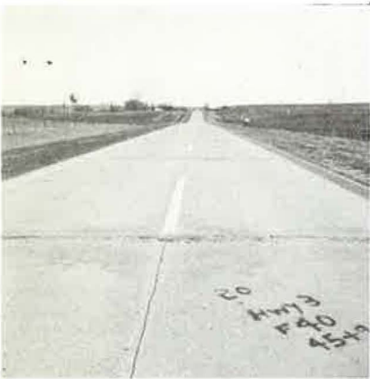
Figure 3. Typical condition of concretes of various ages containing Fayette stone: (a) project 28-10, 27 years old; (b) project 28-11, 24 years old; and (c) project 28-14, 23 years old.
