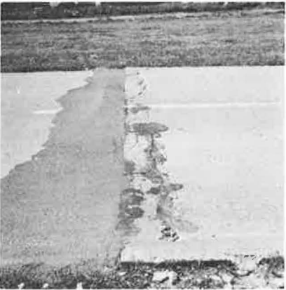
Figure 7. Typical condition of concrete of various ages containing Otis stone: (a) project 53-11, 25 years old; (b) project 52-25, 22 years old; and (c) project 57-38, 18 years old.
