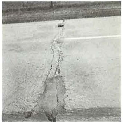
Figure 3. Typical condition of concretes of various ages containing Fayette stone: (a) project 28-10, 27 years old; (b) project 28-11, 24 years old; and (c) project 28-14, 23 years old.
