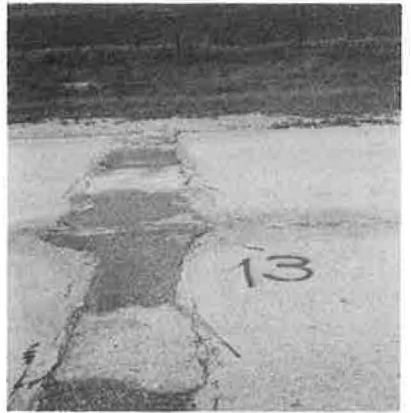
Figure 7. Typical condition of concrete of various ages containing Otis stone: (a) project 53-11, 25 years old; (b) project 52-25, 22 years old; and (c) project 57-38, 18 years old.
