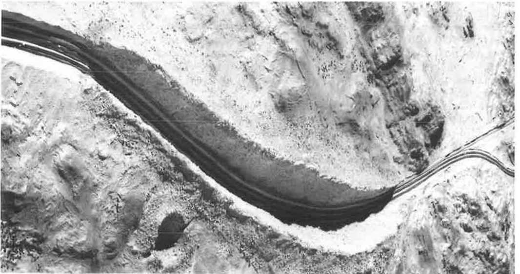
Figure 2. Model of Project Carryall showing drainage crater in relation to roadway excavation.
