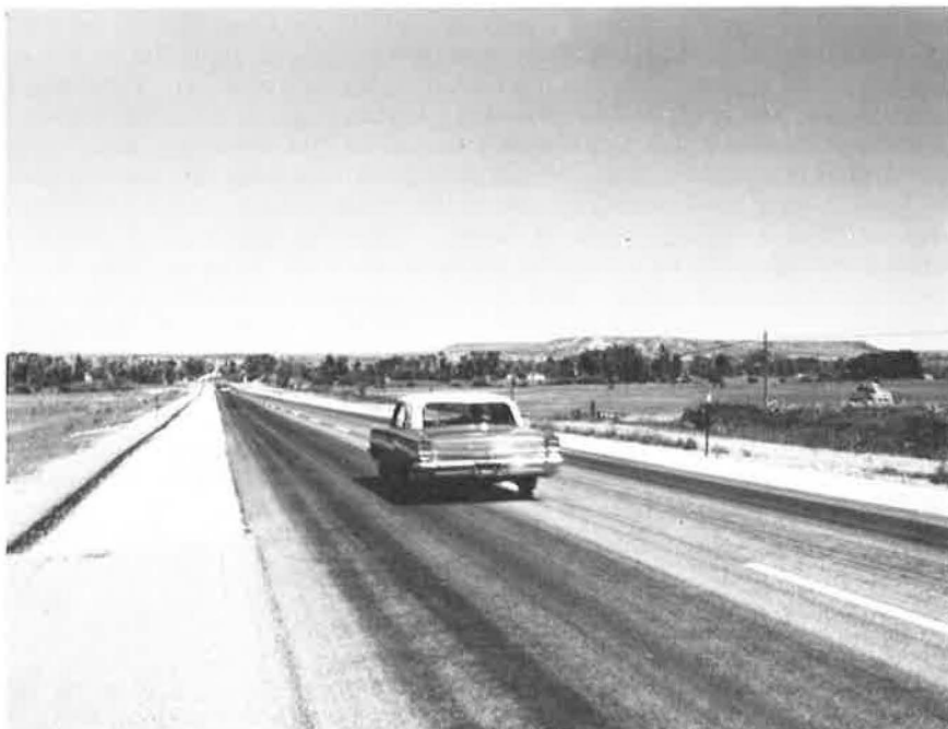
Figure 2. Unsatisfactory (excessively rich) seal coat.
