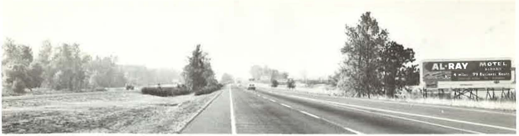
Figure 7. Median planting to delineate curve on I-5 and eliminate headlight glare. Native shrubs added to trees saved during construction.
