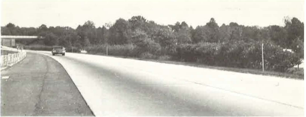
Figure 1. Connecticut Turnpike near Old Saybrooke. Median planting of mixed shrubs provides effective headlight screen.
