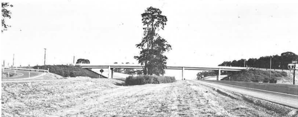
Figure 6. Typical planting of an evergreen ground cover, Bearberry, on interchange slopes too steep to mow mechanically. Native shrubs in median support existing trees, reduce headlight glare and prevent unauthorized crossings (I-5 south of Salem).
