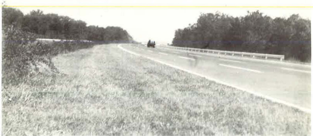
Figure 2. I-80 showing planting of Rosa multiflora in 60-ft median in vicinity of Rockaway, N. J.
