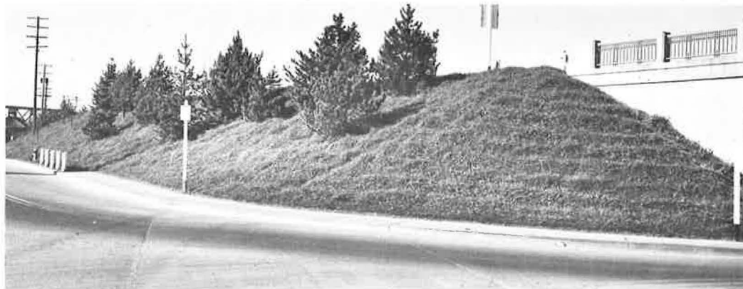
Figure 4. Functional planting on highway slopes. Ground cover reduces maintenance, and pines and crabapples outline curve and screen objectionable old buildings from main roadway (Portland, Ore.).
