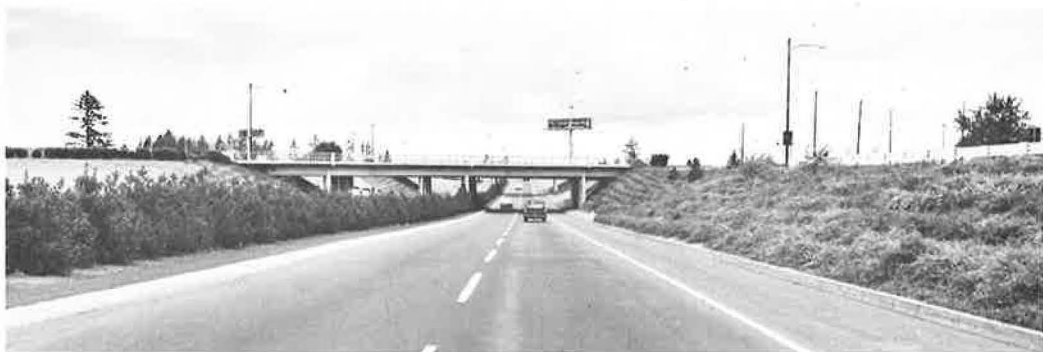
Figure 5. Planting of Oregon Holly in median to eliminate headlight glare. Slopes covered with low-growing ground cover of Bearberry which helps to reduce amount of roadside mowing.
