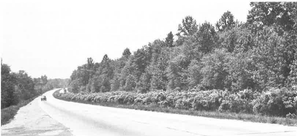
Figure 3. Rosa multiflora planted in 1952 on Virginia Rt. 350, Fairfax Co. Median is 24 ft wide. The Japanese Rose has grown 8 ft high providing a complete screen against headlight glare.
