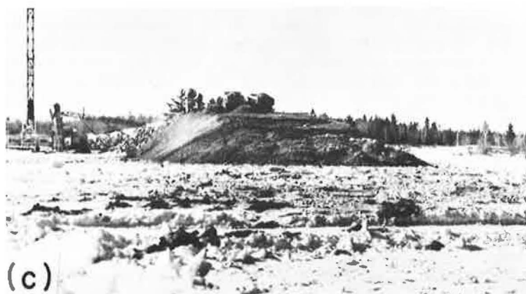
Figure 15. Dynamite blasting ahead of fill: (a) before blast, (b) during blast, and (c) after blast.
