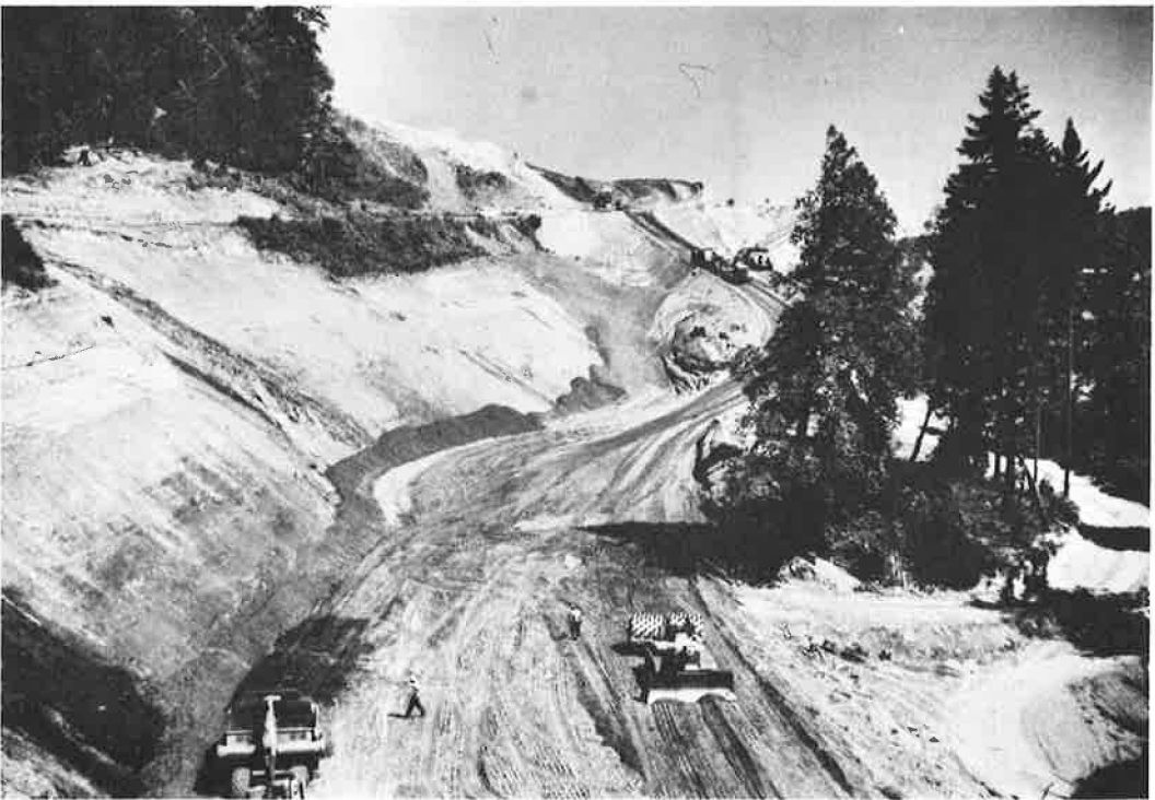
Figure 9. Partially filled longitudinal stabilization trench.
