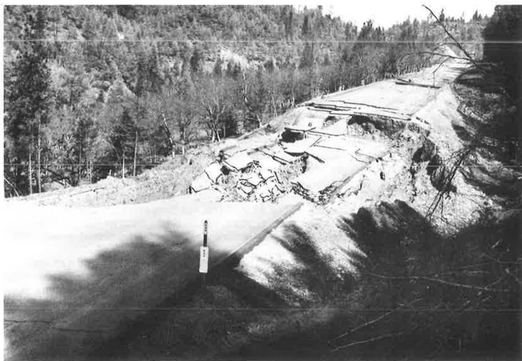
Figure 2. Landslide—fill foundation failure.
