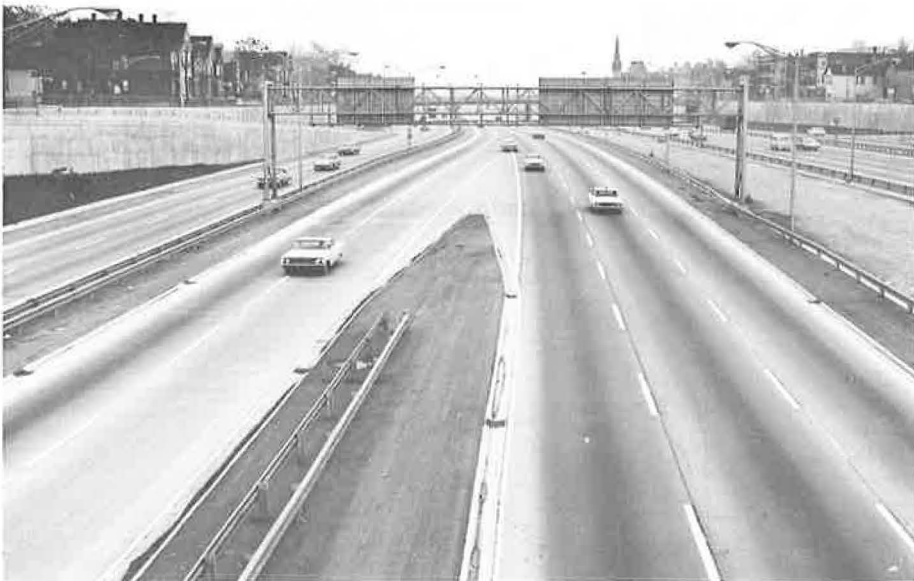
Figure 4. Diverging Terminal of study section with "after" pavement markings.
