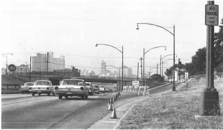
Figure 2. Method of closing North Ave. southbound off-ramp.
