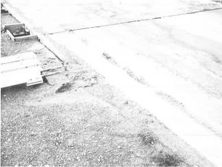
Figure 13. Pumping at U-5, L-5—Nov. 10, 1962.
