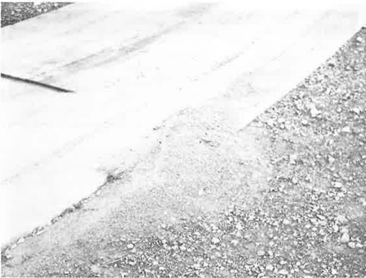
Figure 14. Pumping at bottom of east ramp—Nov. 10, 1962.
