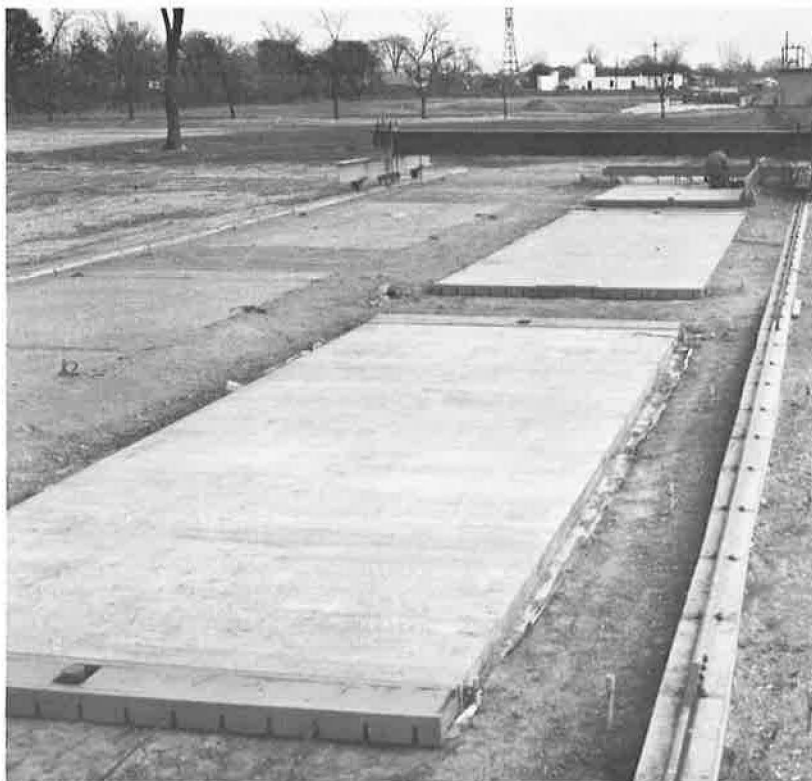
Figure 3. Outdoor test area showing the loading device.
