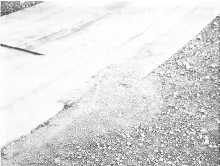
Figure 14. Pumping at bottom of east ramp—Nov. 10, 1962.
