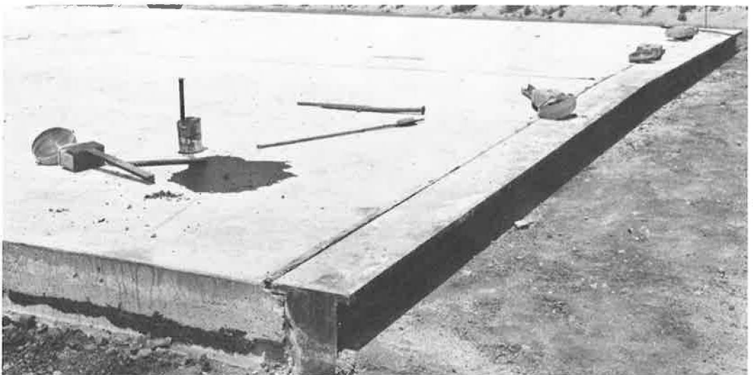
Figure 8. Continuously-reinforced concrete in place against wide-flange beam.
