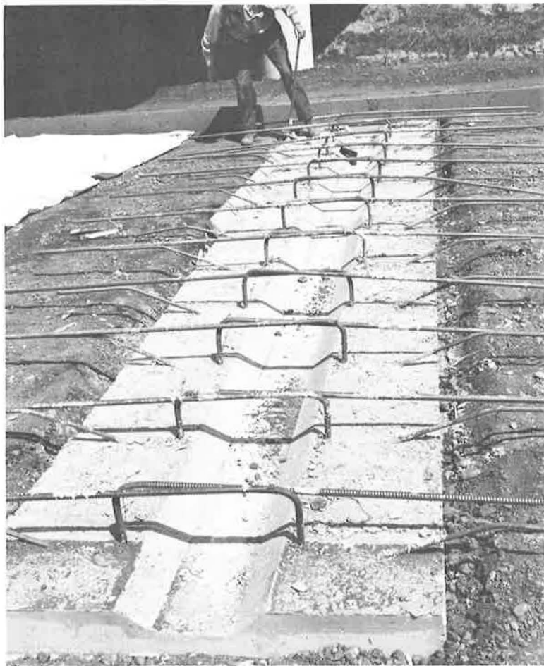
Figure 10. Completed end-anchor lug.
