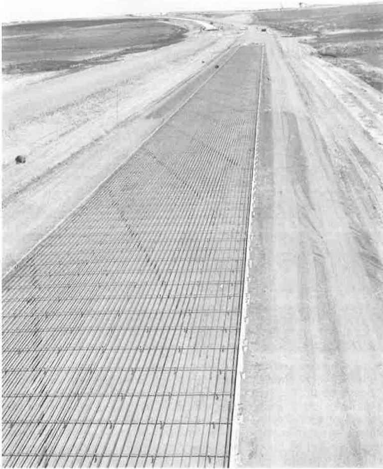
Figure 14. Reinforcing steel in place.
