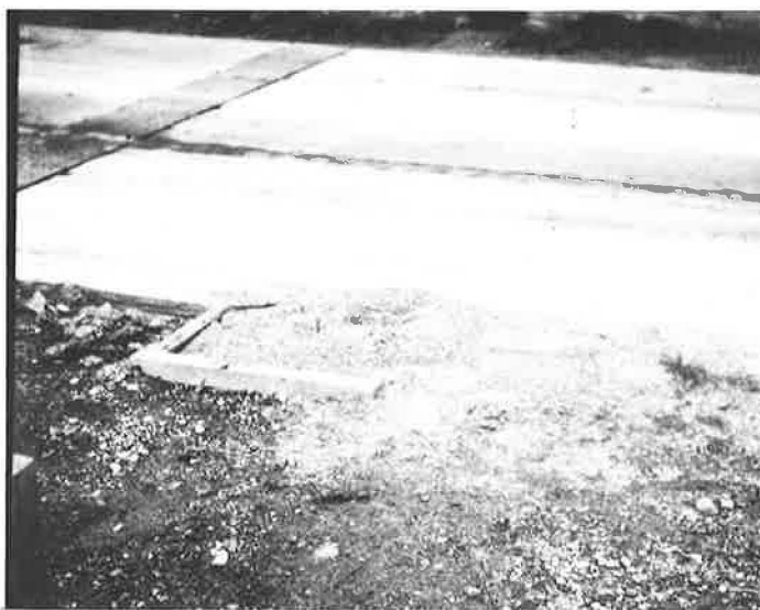
Figure 12. Pumping at U-5, L-5—Oct. 30, 1962.
