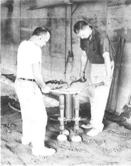
Figure 2. Consolidation of subbase with mechanical tamper.
