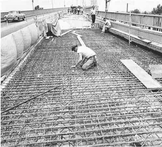
Figure 3. Bayonne Bridge, concrete rehabilitation of full slab depth.
