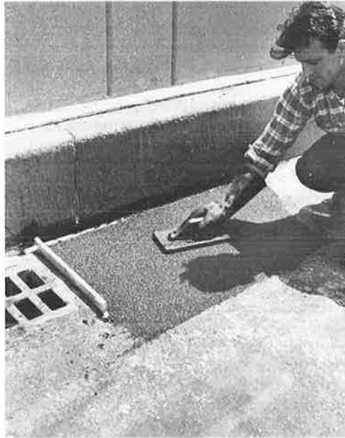
Figure 1. Goethals Bridge, epoxy-coal tar patching compound installed as deck repair.
