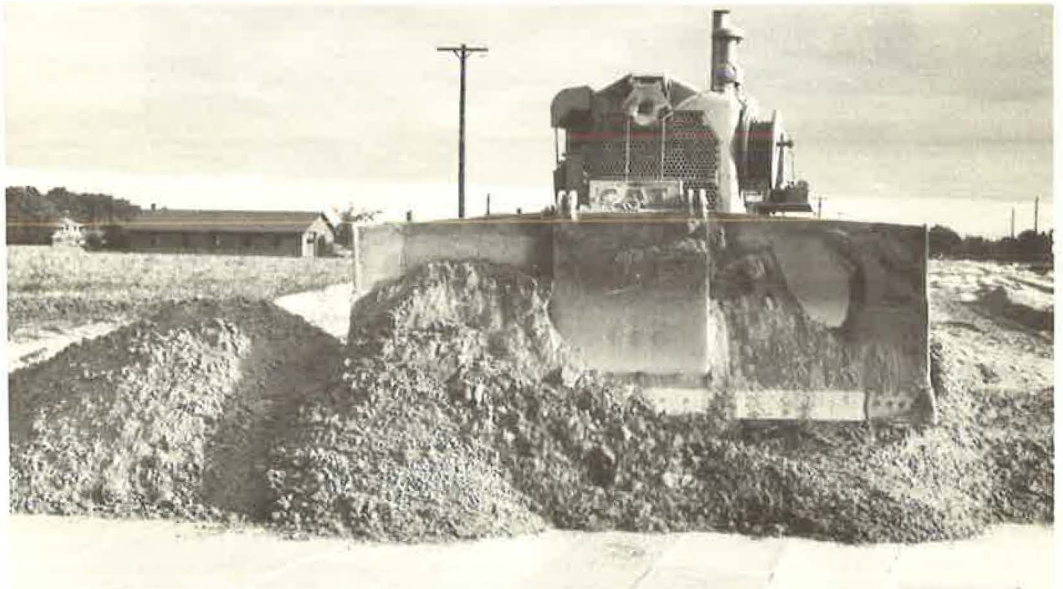
Figure 20. Spreading subbase to 8-in. depth on Styrofoam insulating layer in Michigan.
