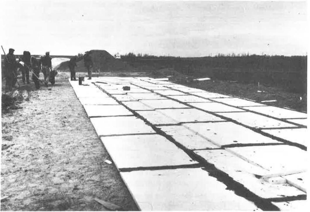
Figure 2. Partially completed section 2 showing two layers of foam plastic.
