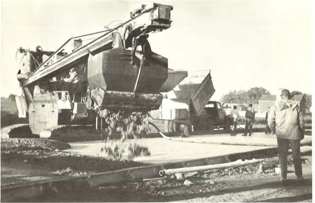
Figure 19. Placement of concrete on Styrofoam insulating layer in Iowa.
