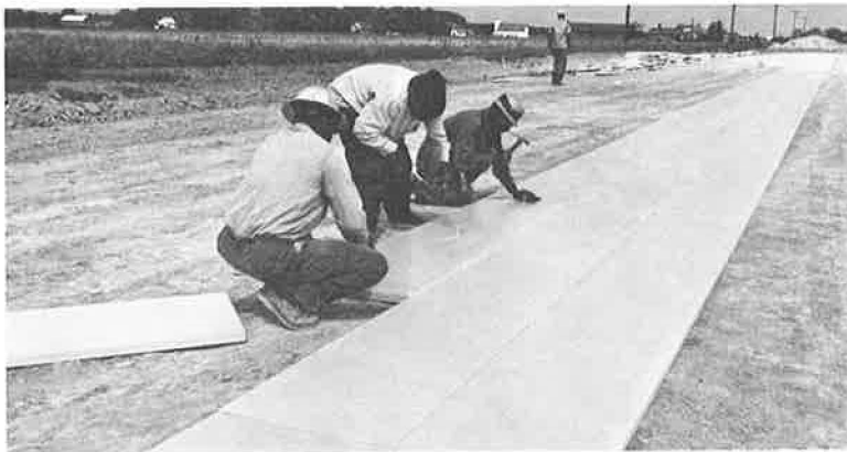
Figure 17. Styrofoam insulating layer being placed on graded subgrade for flexible pavement in Michigan.
