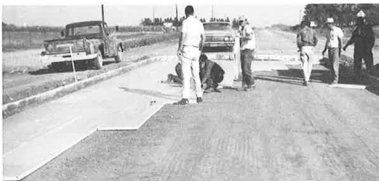
Figure 18. Placement of Styrofoam insulating layer for concrete pavement in Iowa.
