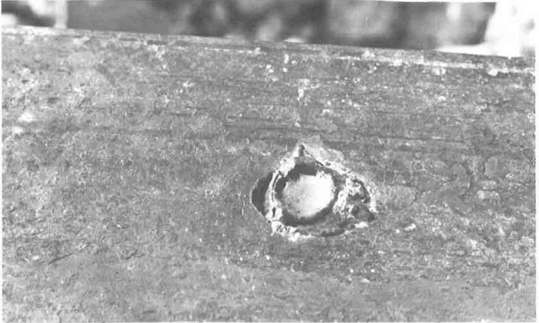
Figure 13. Stud failure in specimen 2-C.
