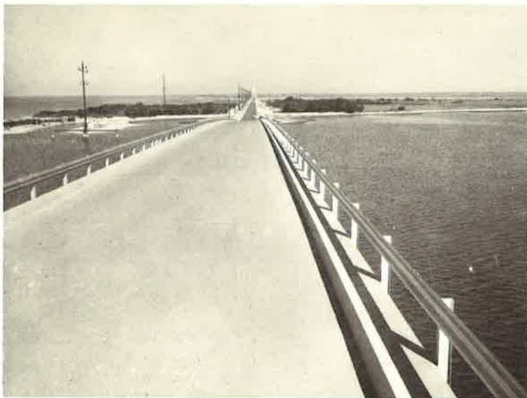
Figure 1. Dauphin Island bridge.
