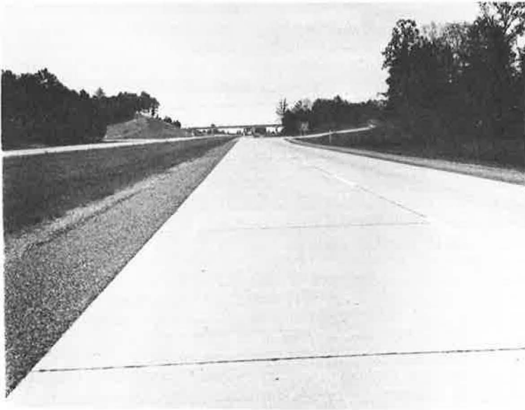
Figure 3. Section of concrete paving containing fly ash.
