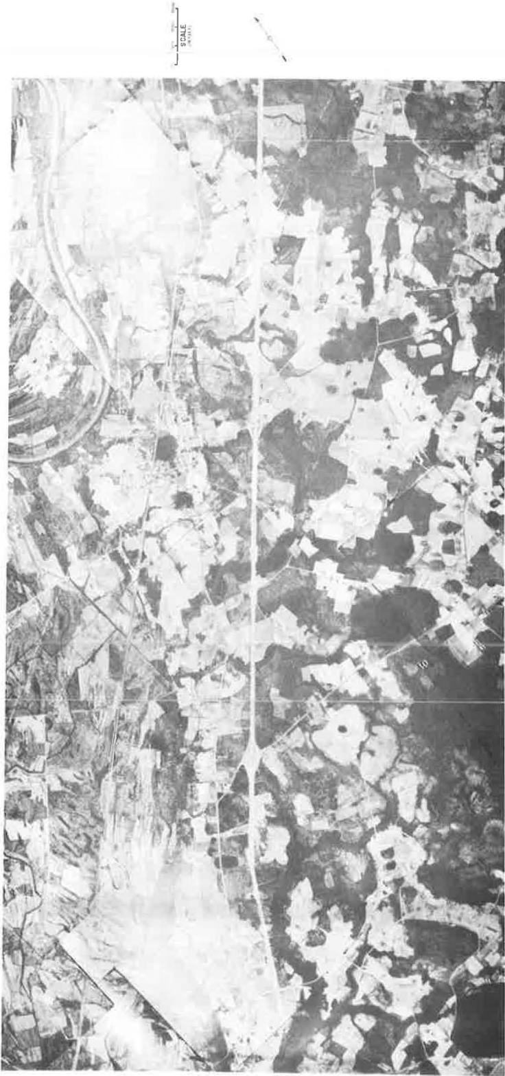
Figure 4. After-period aerial view of I-95 site.
