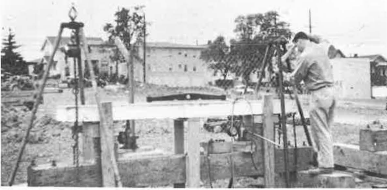
Figure 17. Making measurements on one of the control test beams.
