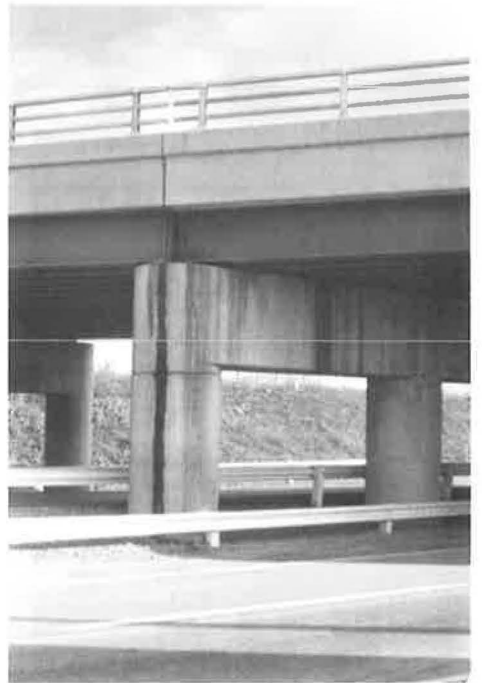
Figure 23. Straining of concrete.
