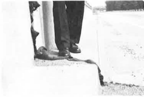
Figure 24. Accumulations of incompressibles, "elephant earing."
