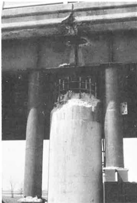
Figure 19. Salt brine corrosion.
