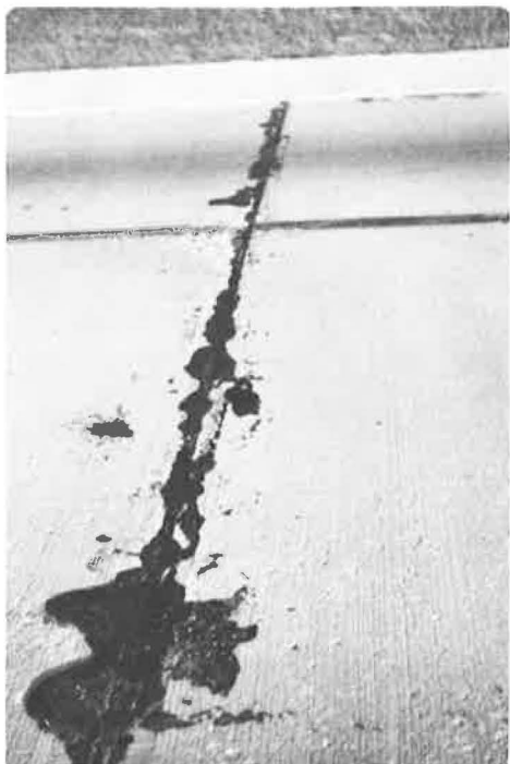
Figure 5. Repeated resealing.
