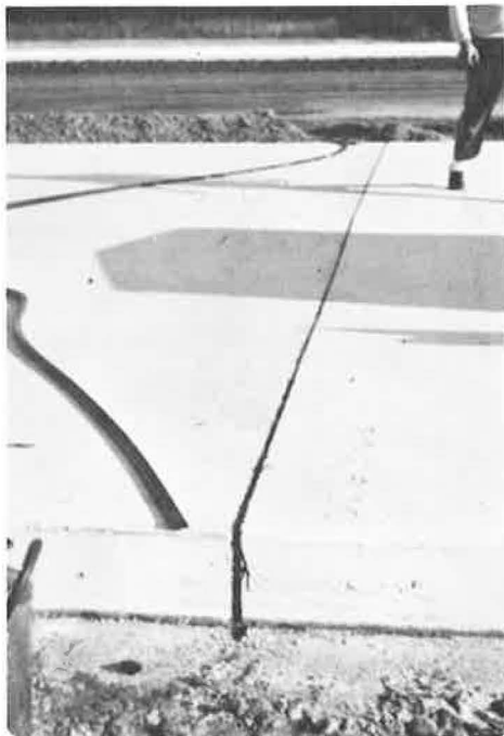
Figure 15. Pavement edge sealing.
