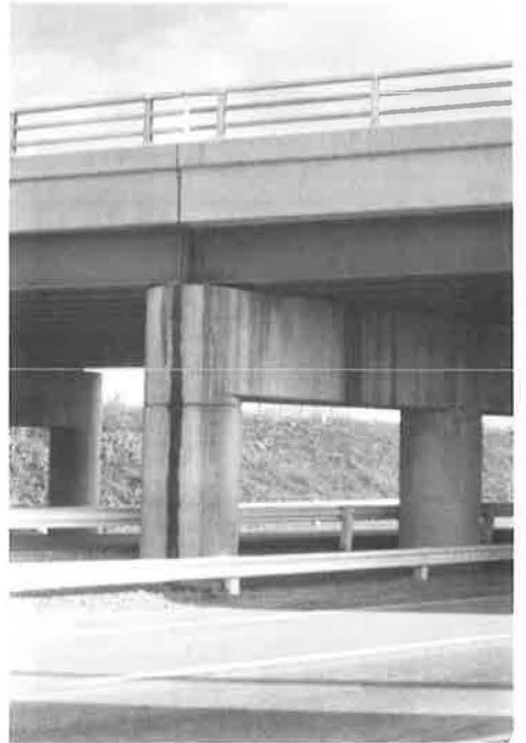
Figure 23. Straining of concrete.
