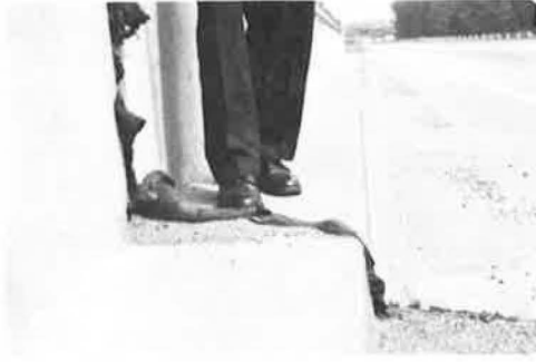
Figure 24. Accumulations of incompressibles, "elephant earing."
