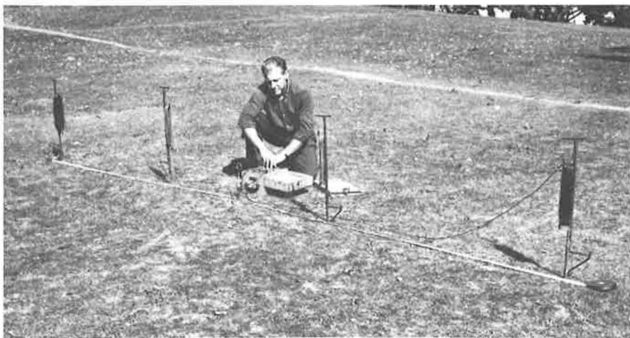
Figure 1. Resistivity instrument as set up to take readings.
