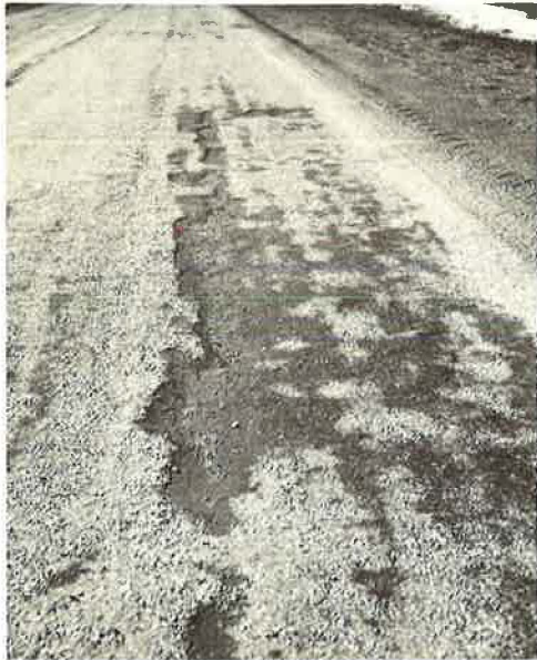
Figure 12. Surface damage due to failure of single bituminous seal, Iowa 37.
